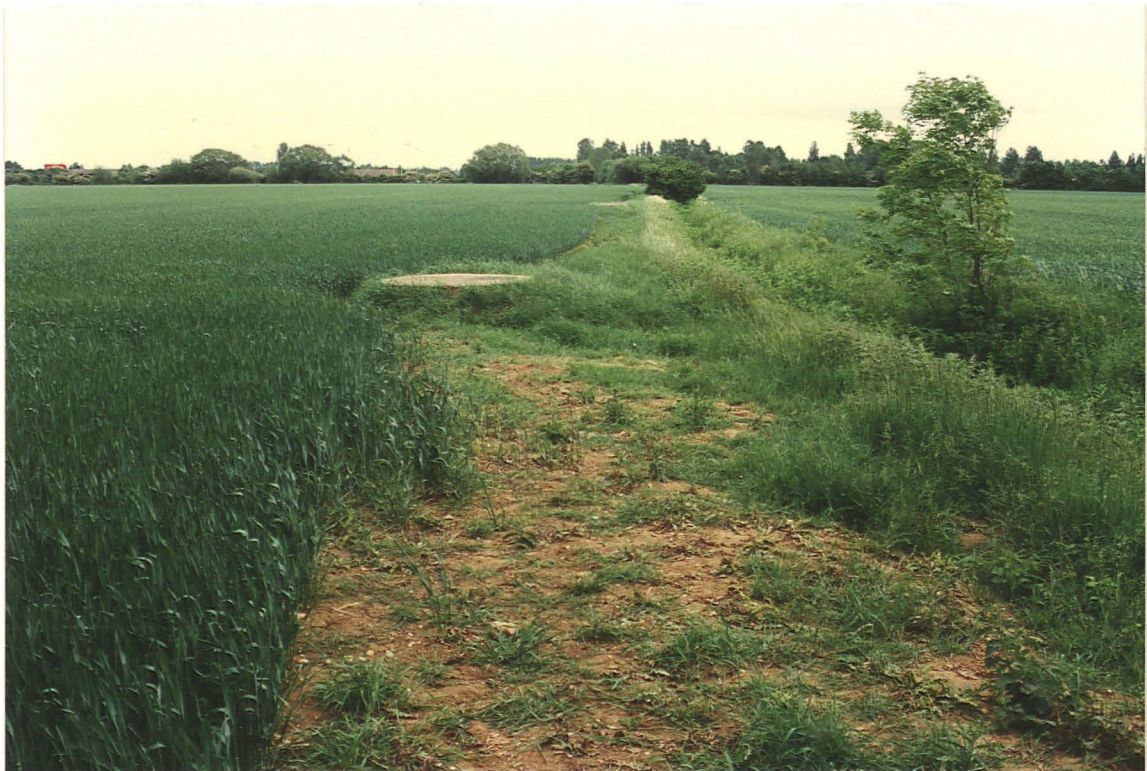
Pl. 4 The southern boundary of Field 2, with raised sewer inspection points visible. Looking east.
