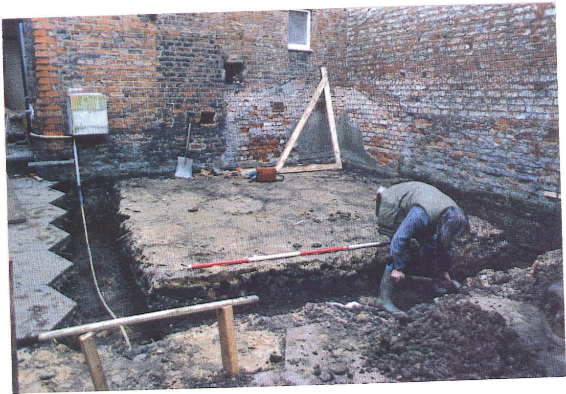
PI.1 General view of site, excavating remainder of footings, looking SE.
