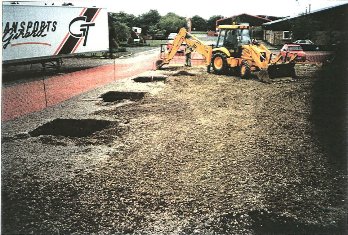
Plate 1 General View of Development, looking east
