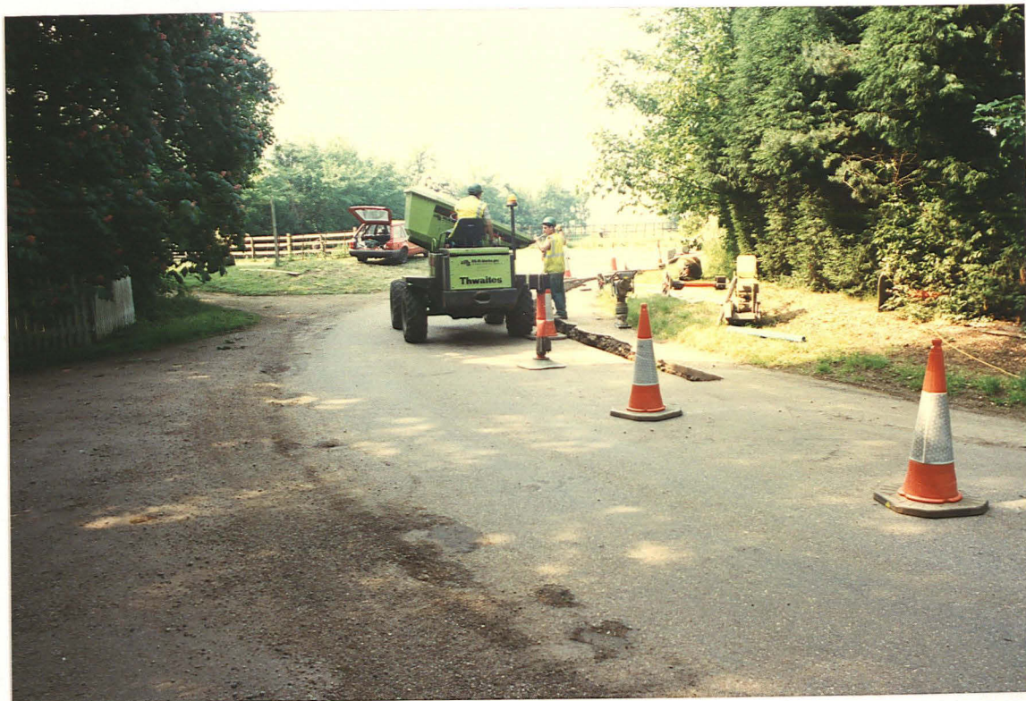
Pl. 10 Junction of the road through Bloxholm with a farm track thought to fossilise the route of King Street. Post-medieval feature 12 was beside the dumper. Looking SW.
