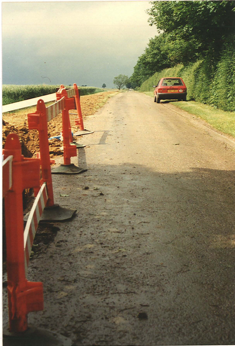
Pl. 6 View north along Bloxholm road from Springwell Plantation.
