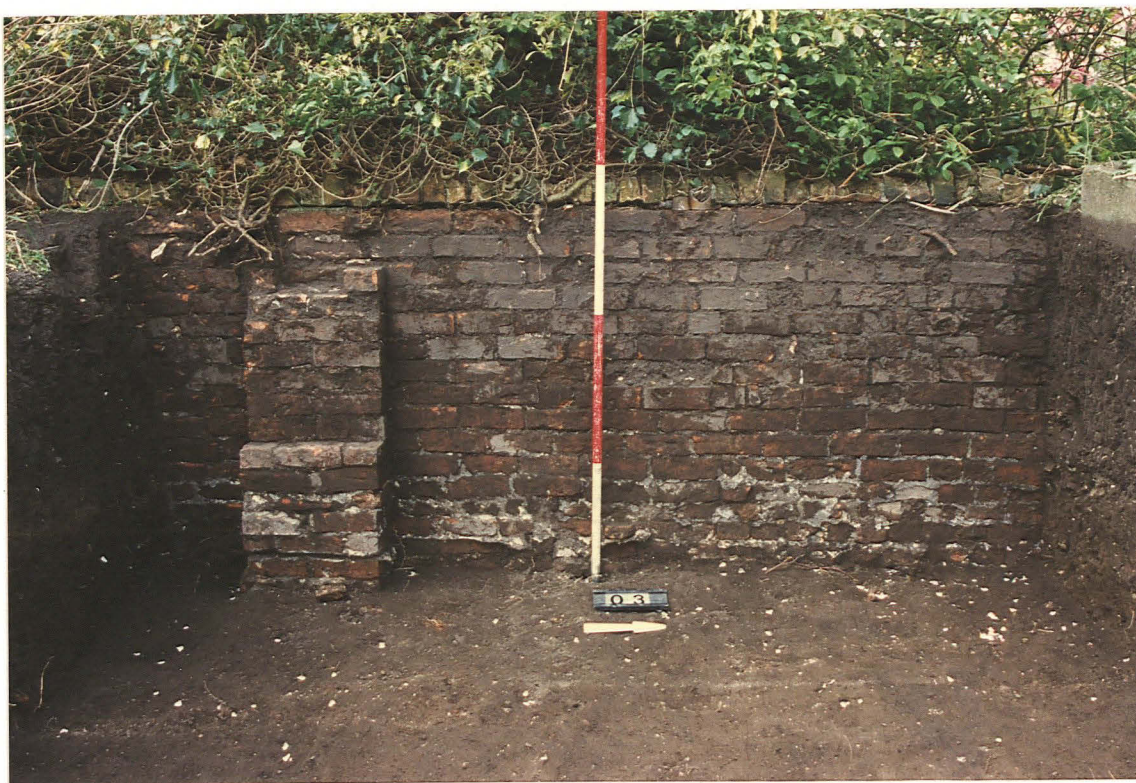
Pl.19 E-facing elevation of present west boundary wall. Looking W. Scale 2m.
