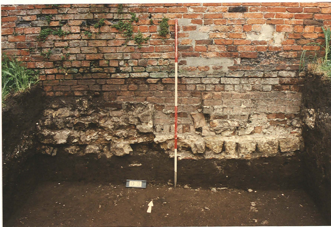
Pl.18 S-facing elevation of present building and foundations. Looking N. Scale 2m.
