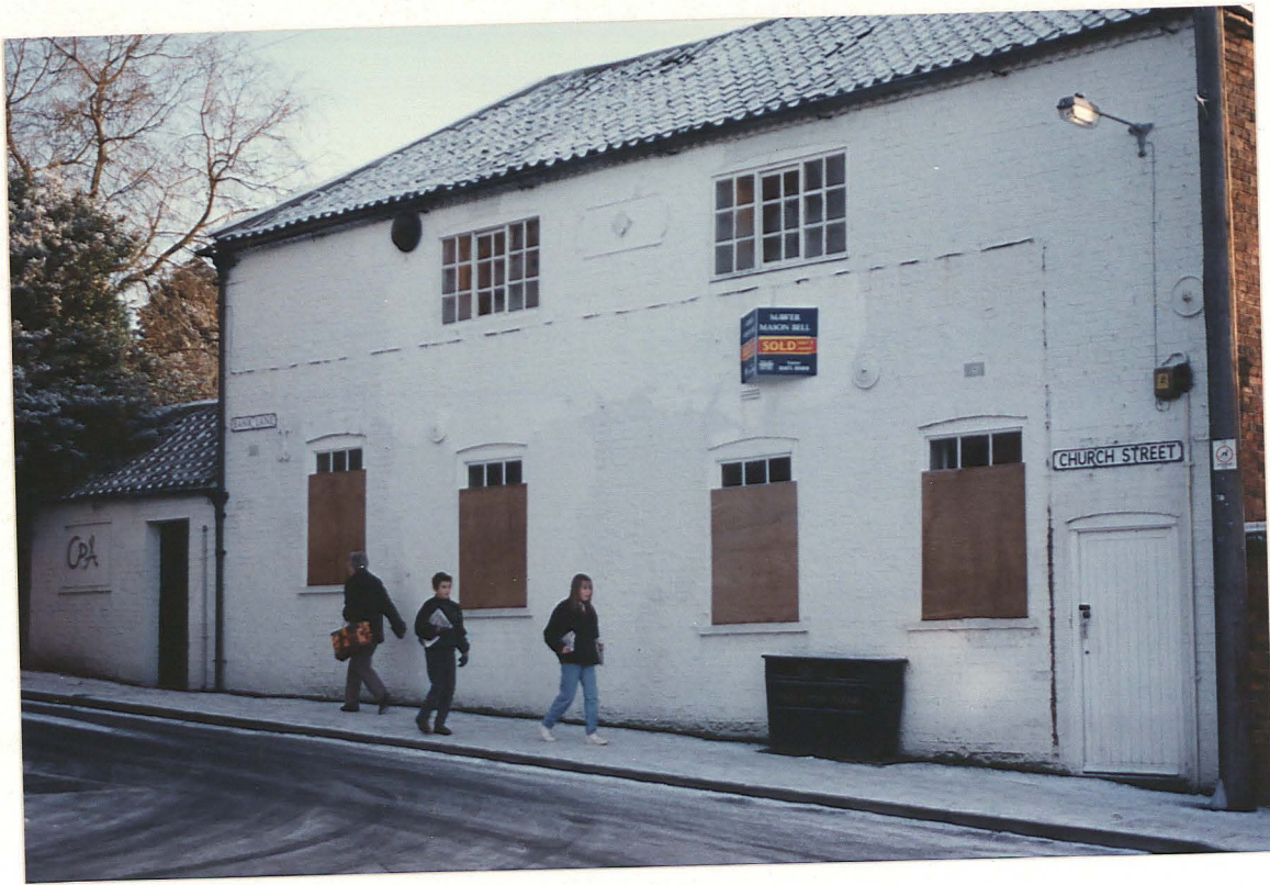
PI.1 View of front elevation of former British Legion Hall, Bank Lane. Looking SE.
