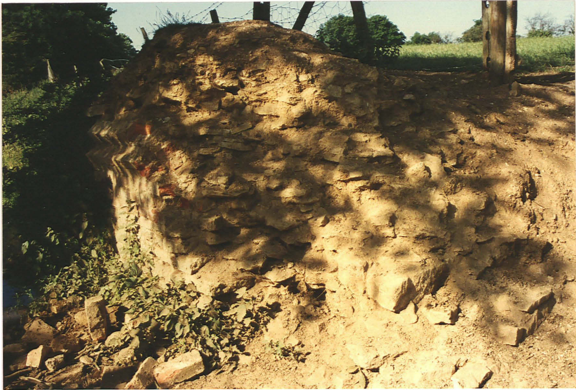
Pl. 26. Western side of demolished stone bridge 41 (looking west). Note the brick arch facing.
