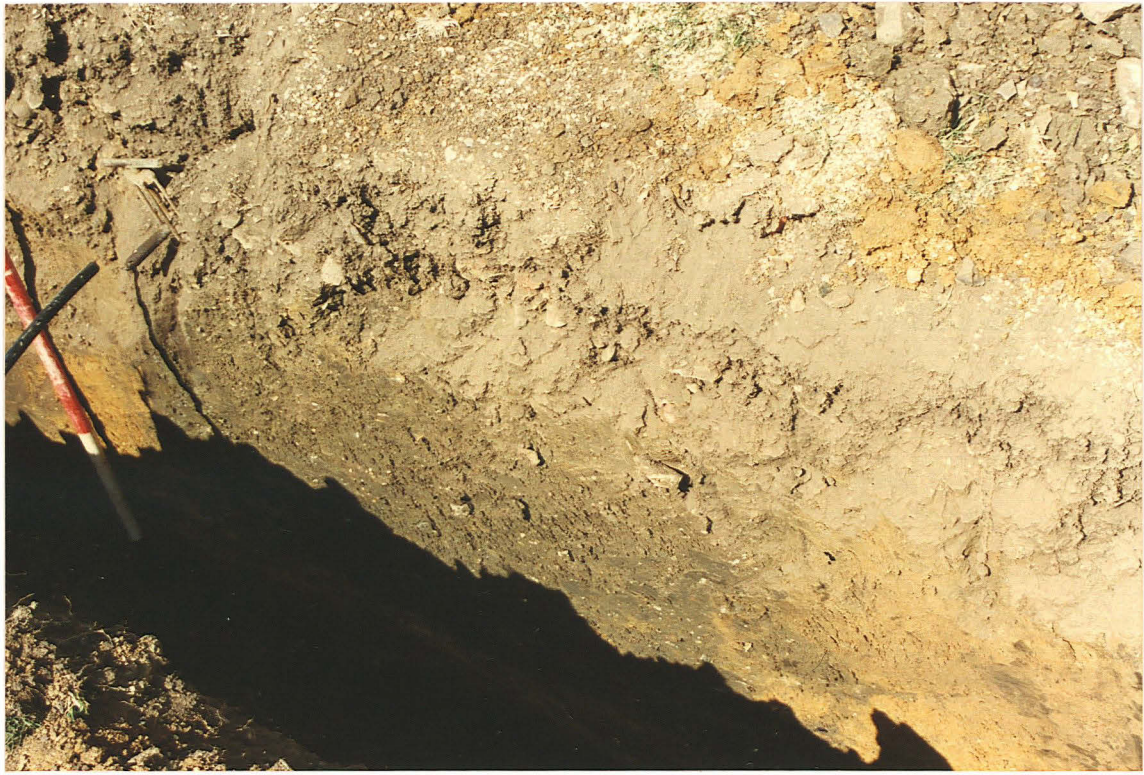
Pl. 3. Dark soil backfill of Ditch 1, showing position of water supply pipe (looking east; scale divisions 0.5m).
