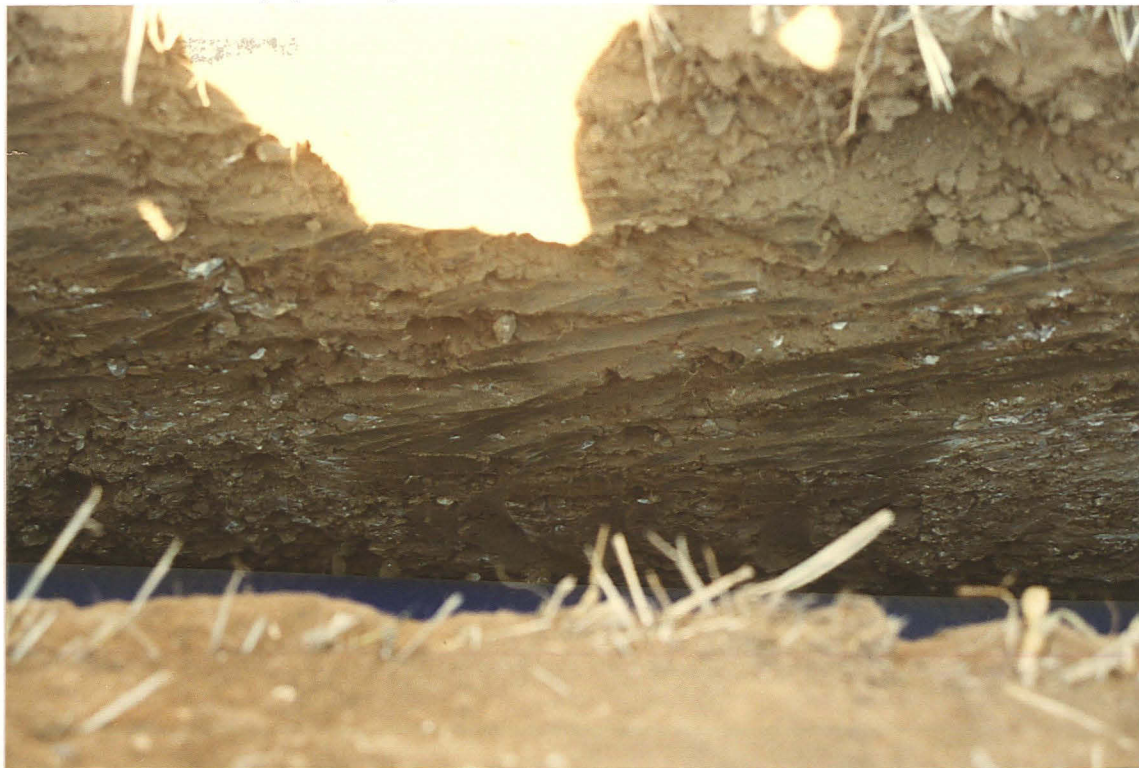
PI. 31. Feature 43: a vertical-sided trench backfilled with brown clay, seen in the pipe trench face. This may have been a land drain, with the pipe deeper than the monitored trench.
