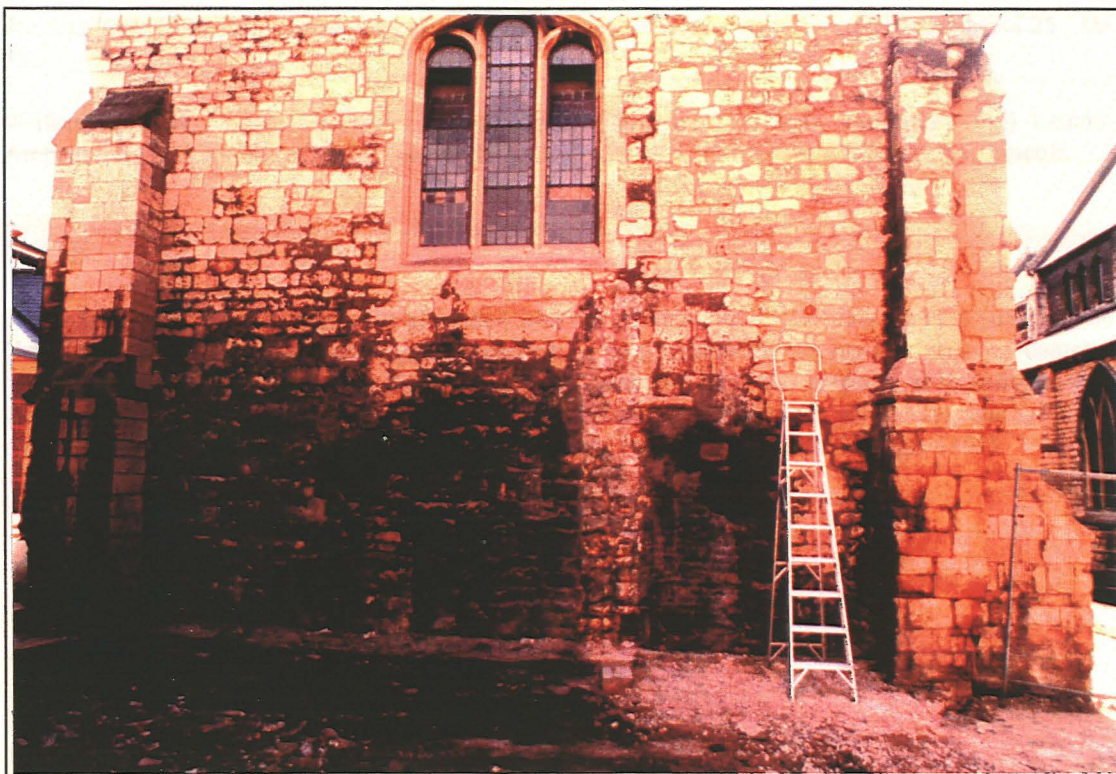
Fig. 3: View looking east showing west gable after the removal of the archway abutment (also see Fig. 6).
