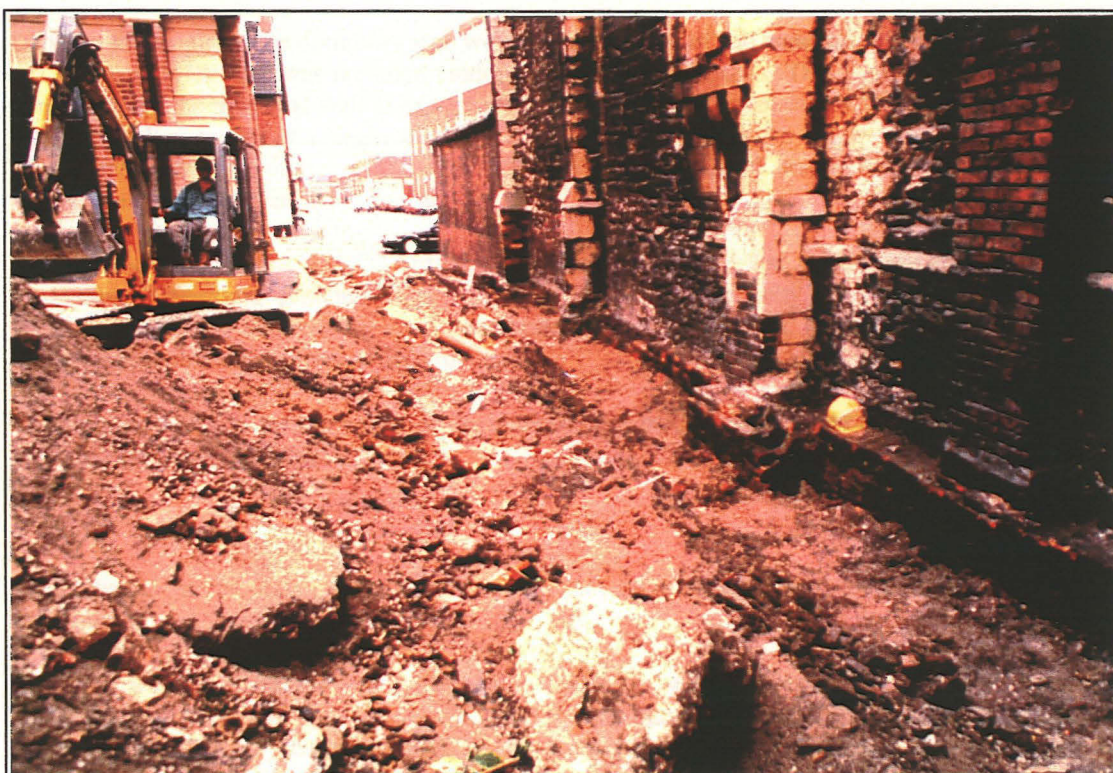
Fig. 2.: Reducing ground level on the northern side of Greyfriars. The brick 'ventilation' wall lies at the base of the Greyfriars elevation (also see Fig. 5).
