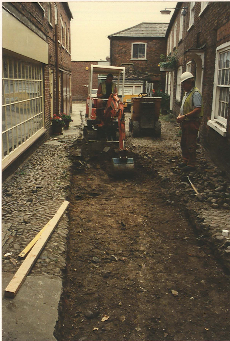
Pl. 3 Lindsey Court, view south, clearance of tarmac in preparation for resurfacing. No visible archaeological remains.
