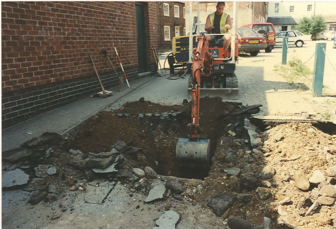
Pl. 4. Excavation of second trench with mini-excavator east of library, view north.
