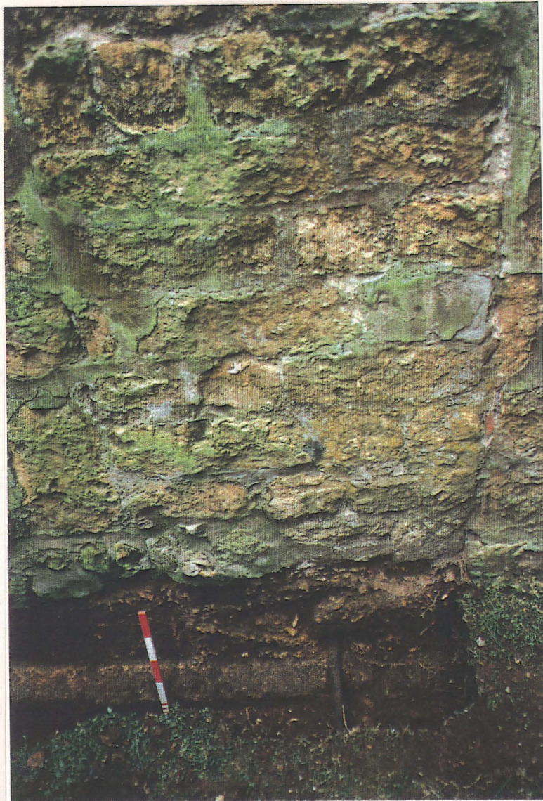
Pl. 3 Chamfered plinth runs uninterrupted beneath blocked door.
