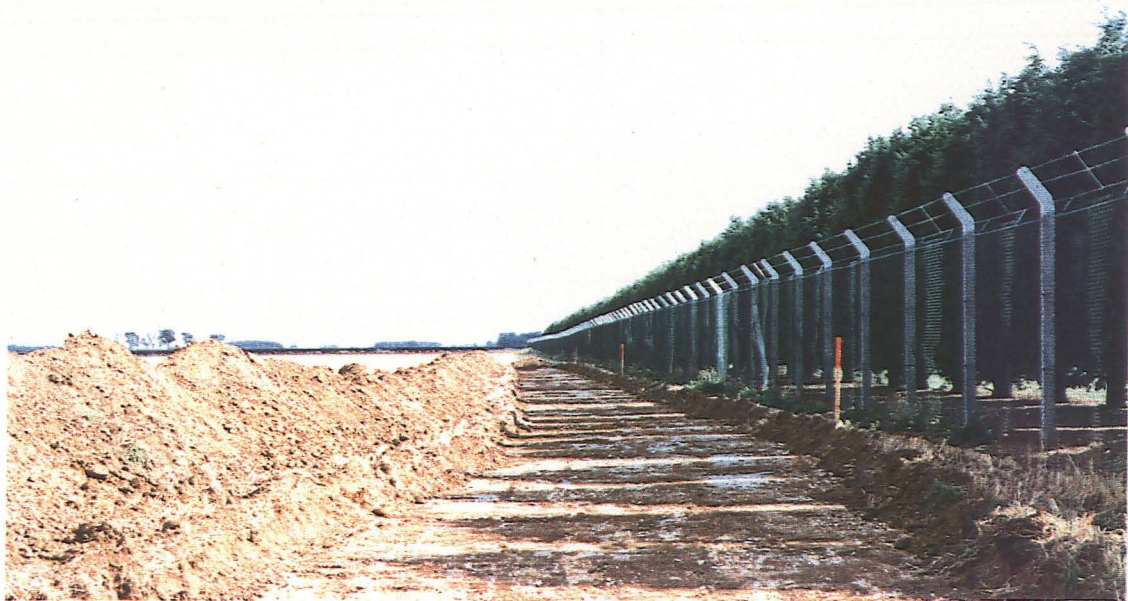
P2 Access road looking east, adjacent to RAF Waddington
