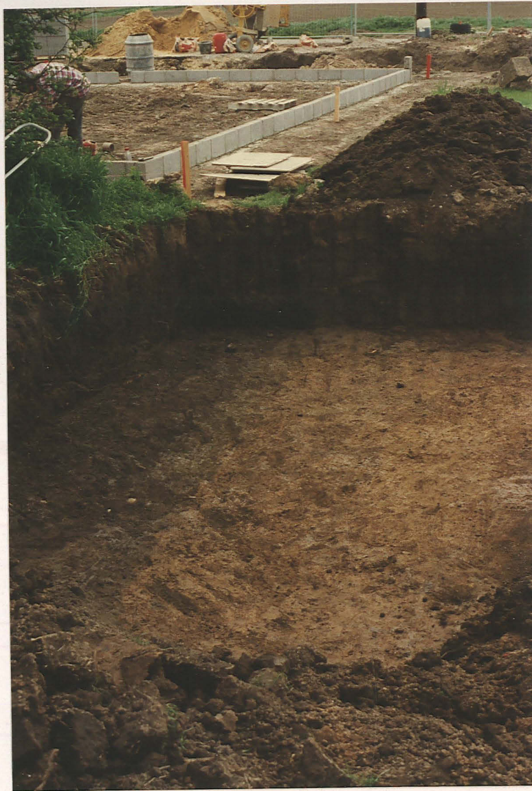
PI. 23 Septic tank trench. Ditch 56 (left) cutting ditch 60 (trench edge).
