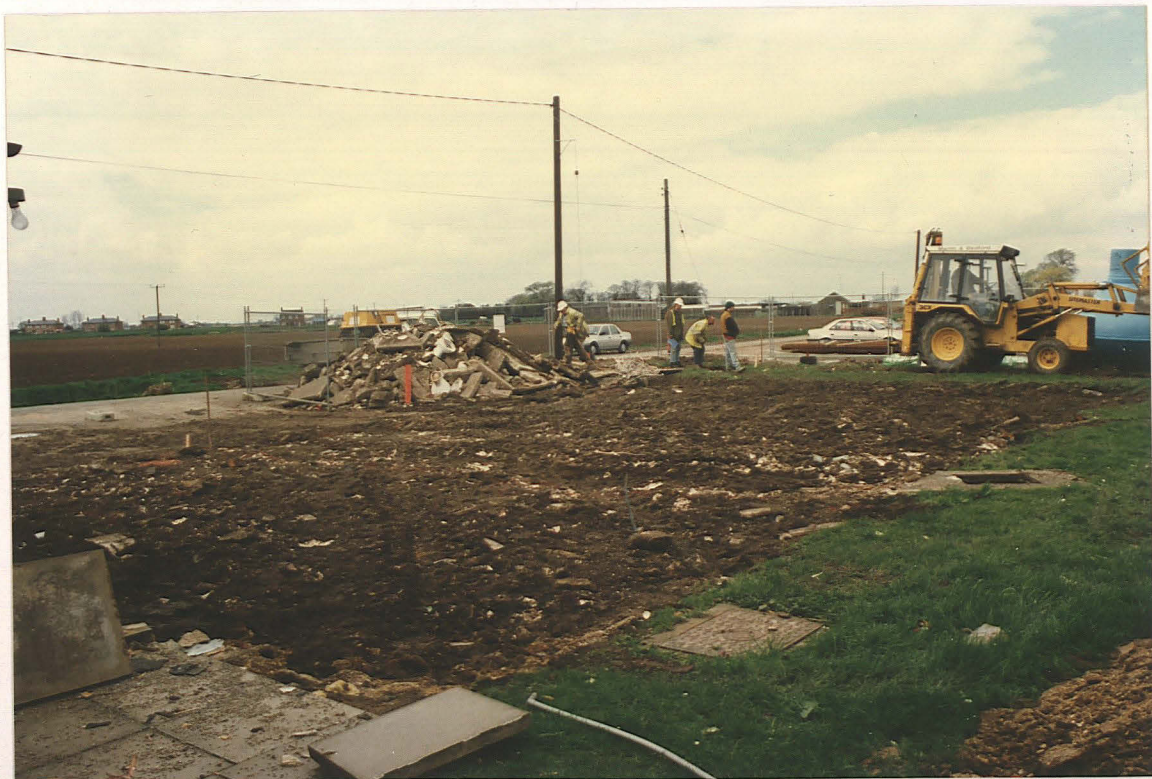
PI. 24 Site of new classroom foundations.
