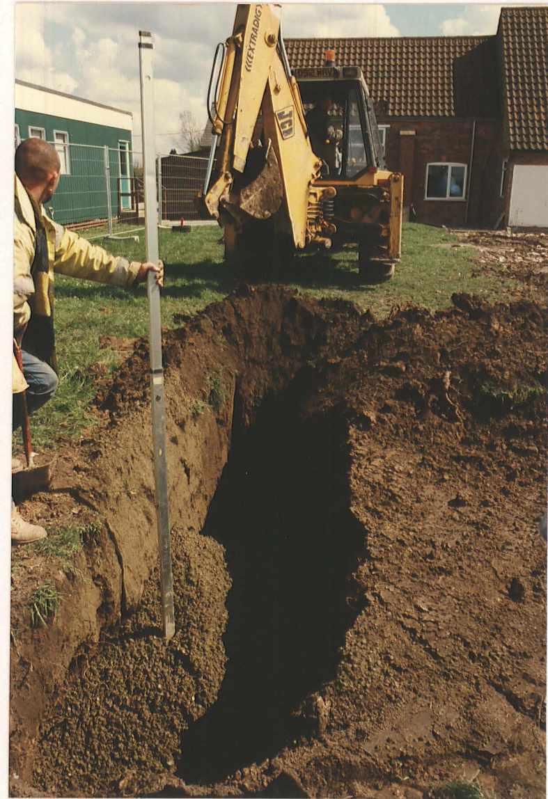
Pl. 25 Temporary shoring in classroom foundation trench.
