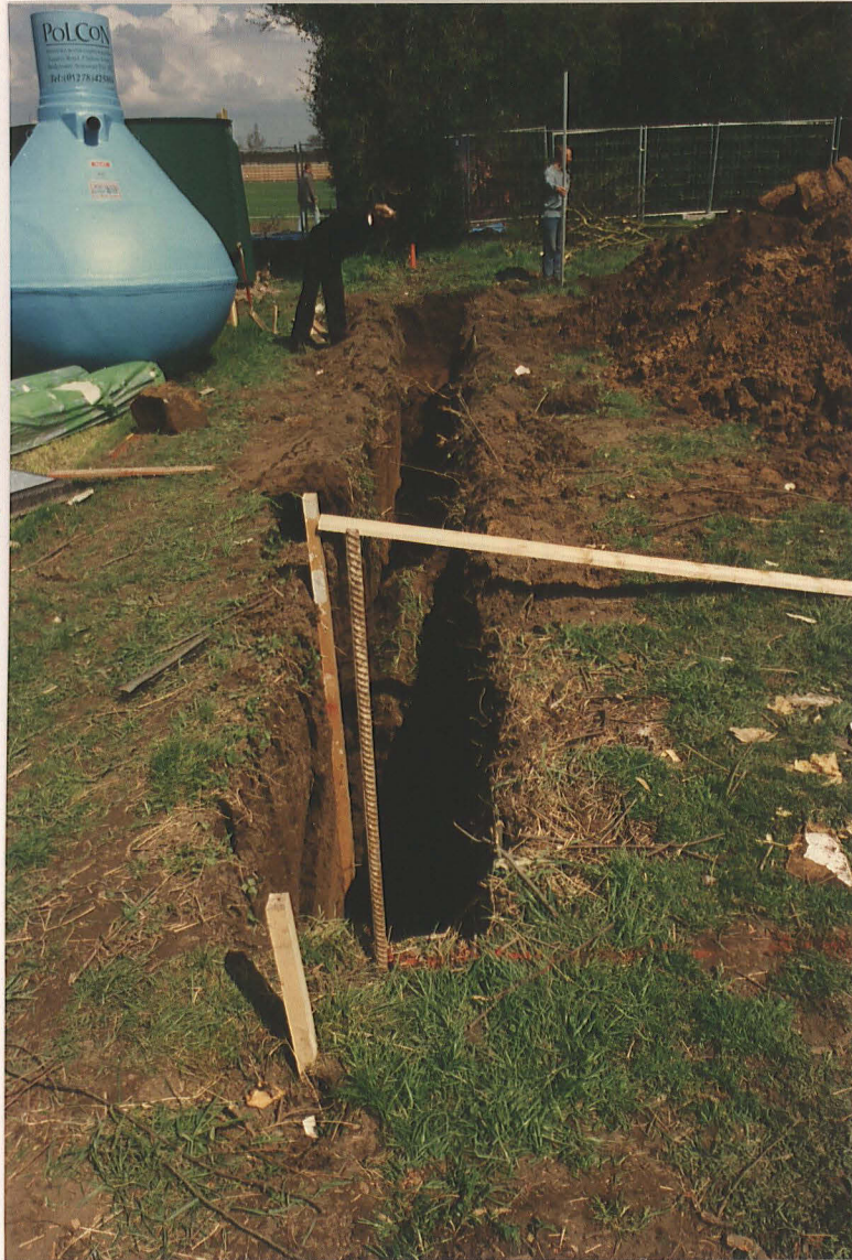
Pl. 25 Temporary shoring in classroom foundation trench.
