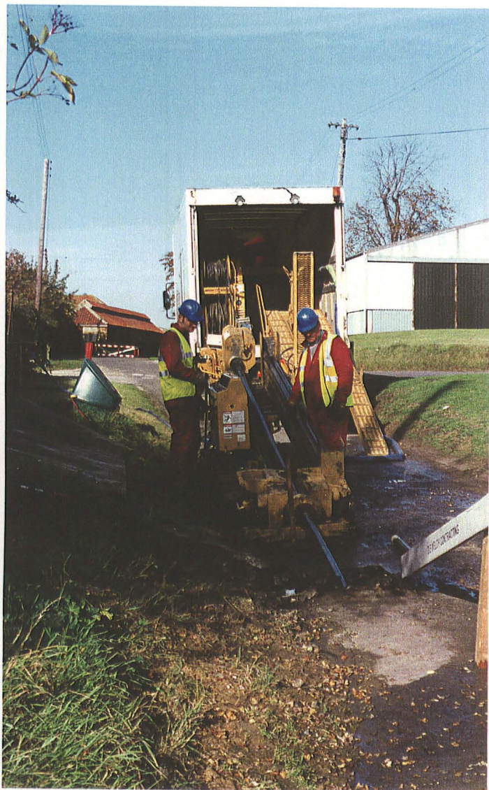
Plate 1: General shot of thrust bore operation at Access Pit 4
