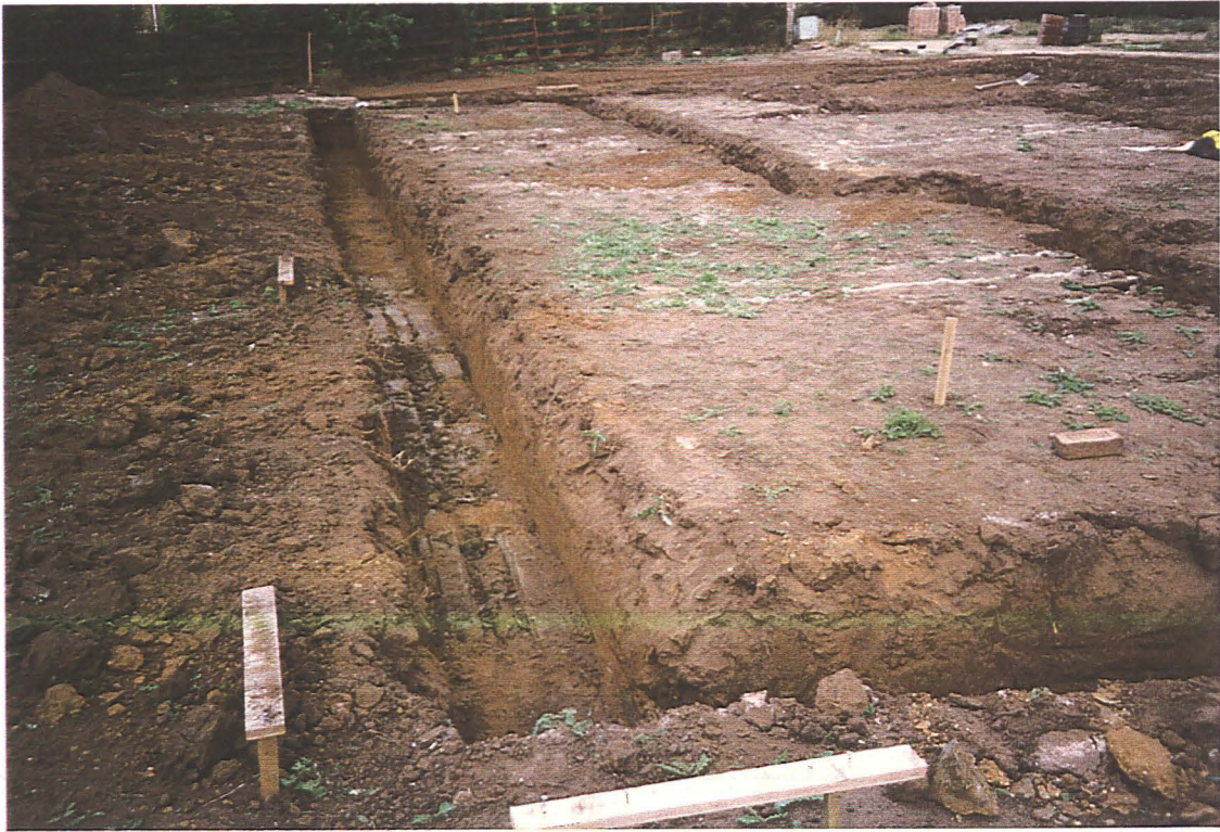
Plate 1: General Site View
