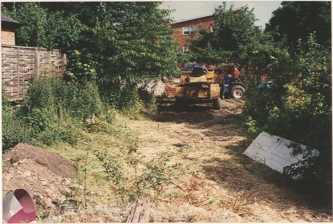
Pl. 1. Location of proposed outbuilding, looking north.
