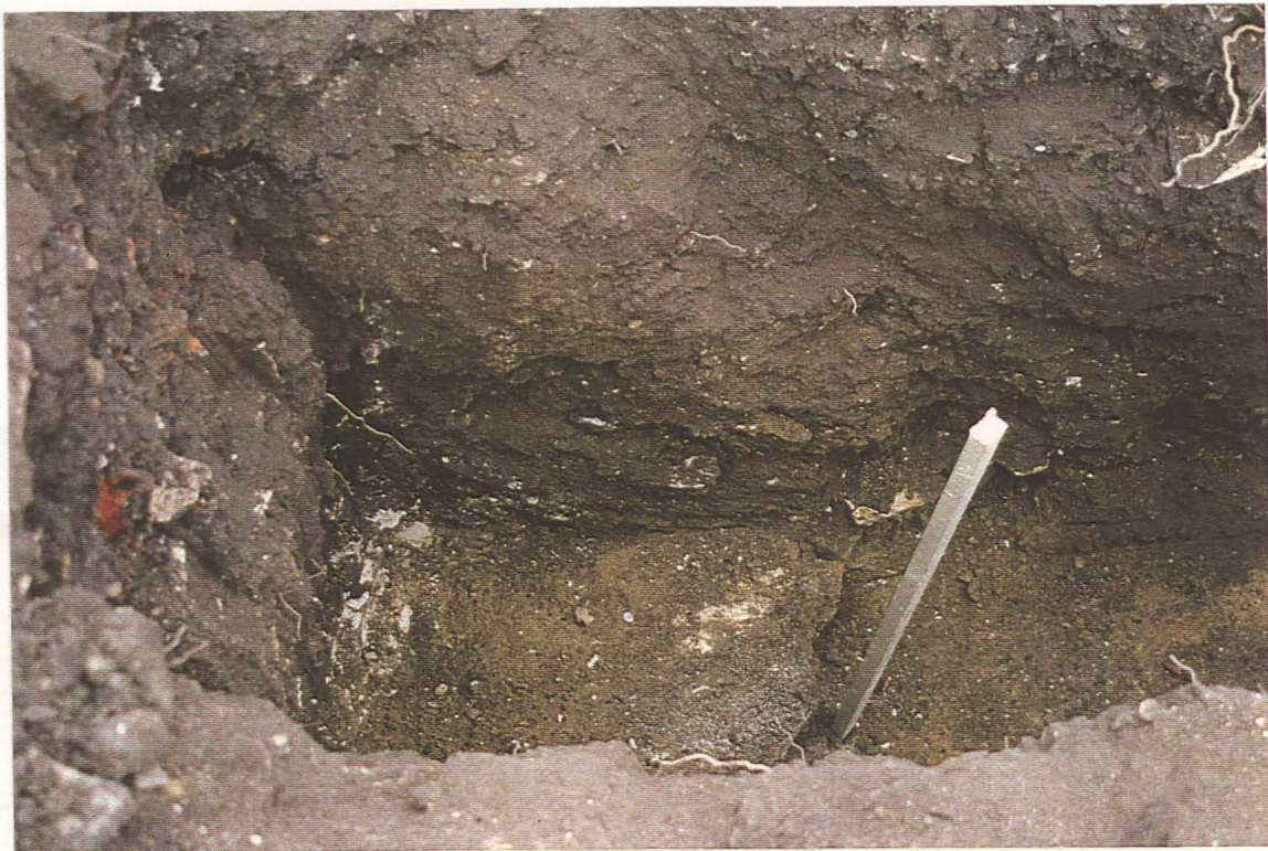
Pl. 19. Kitchen/conservatory (east) foundation trench. Possible wall 114, looking west.
