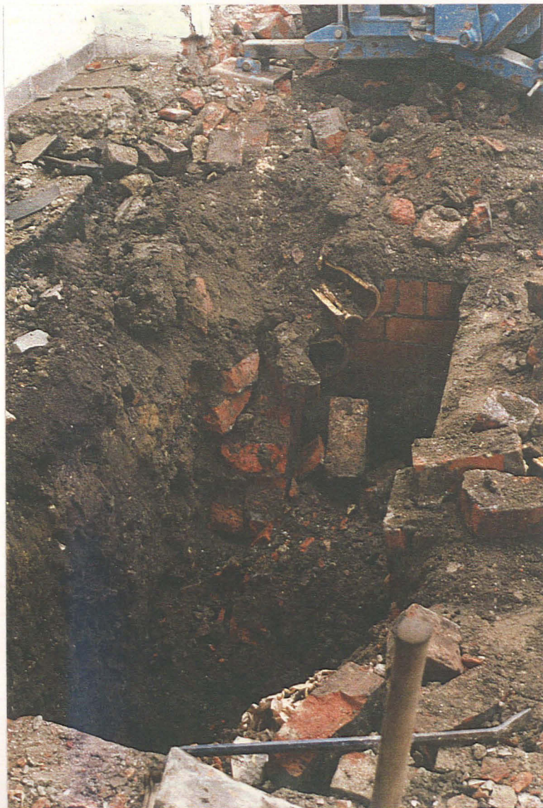
Pl. 24. West trench of house. Brick inspection chamber 44 with drain 58 visible amongst the rubble during excavation. Looking north.
