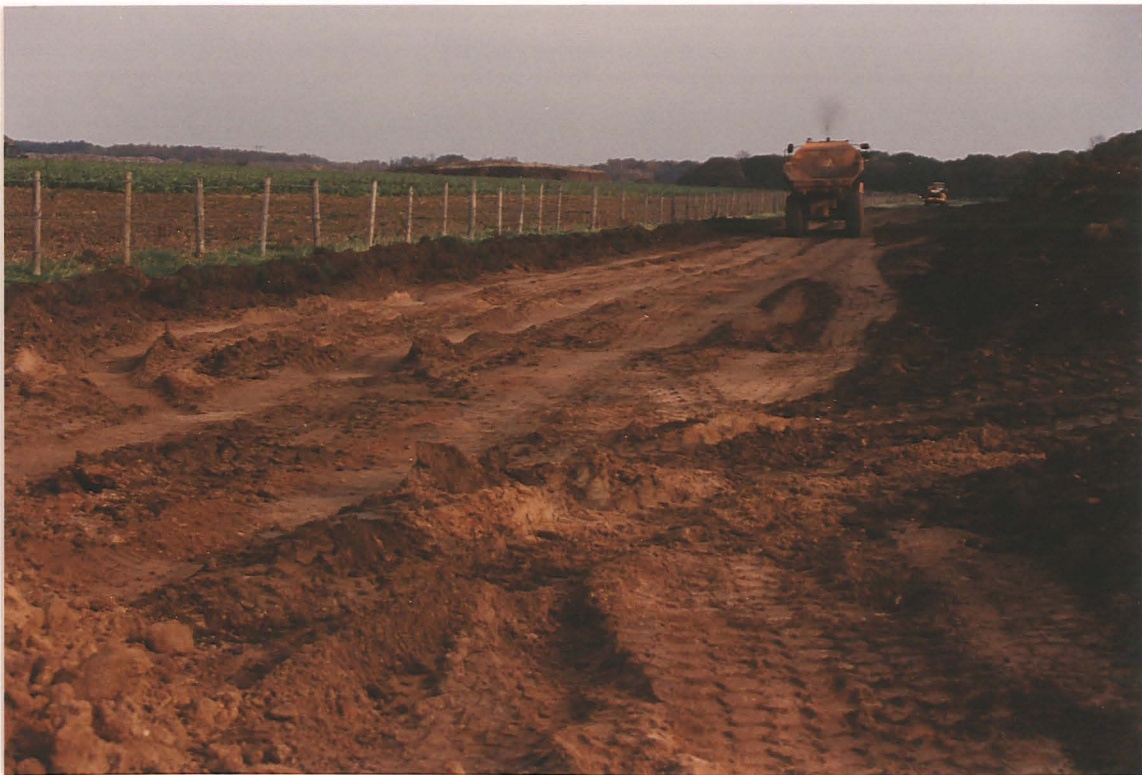
Pl. 29 Machine trampling completely obscured the unmonitored soil horizon on the site of the perimeter bund (looking NE towards Fox Covert).
