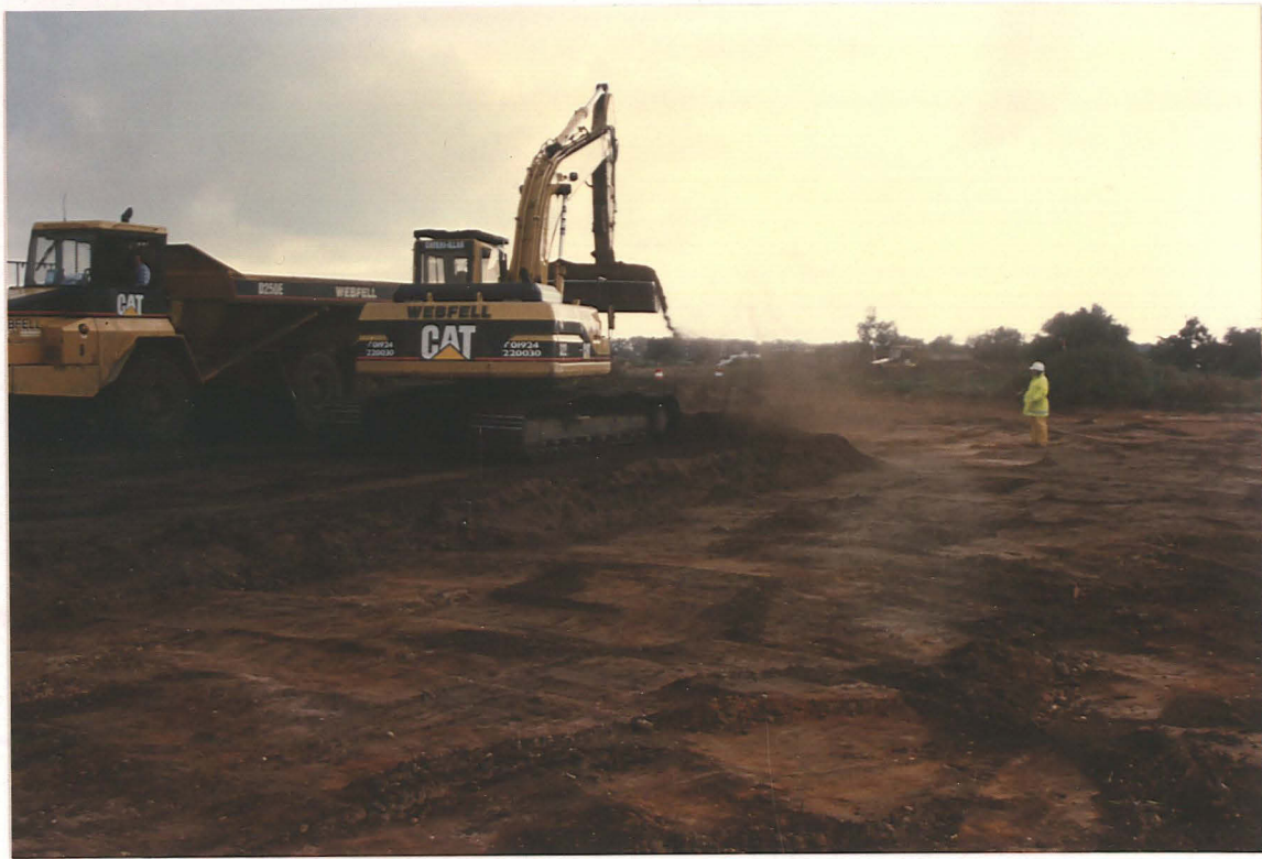
Pl. 2 The method used to remove topsoil, with archaeological monitoring in progress.
