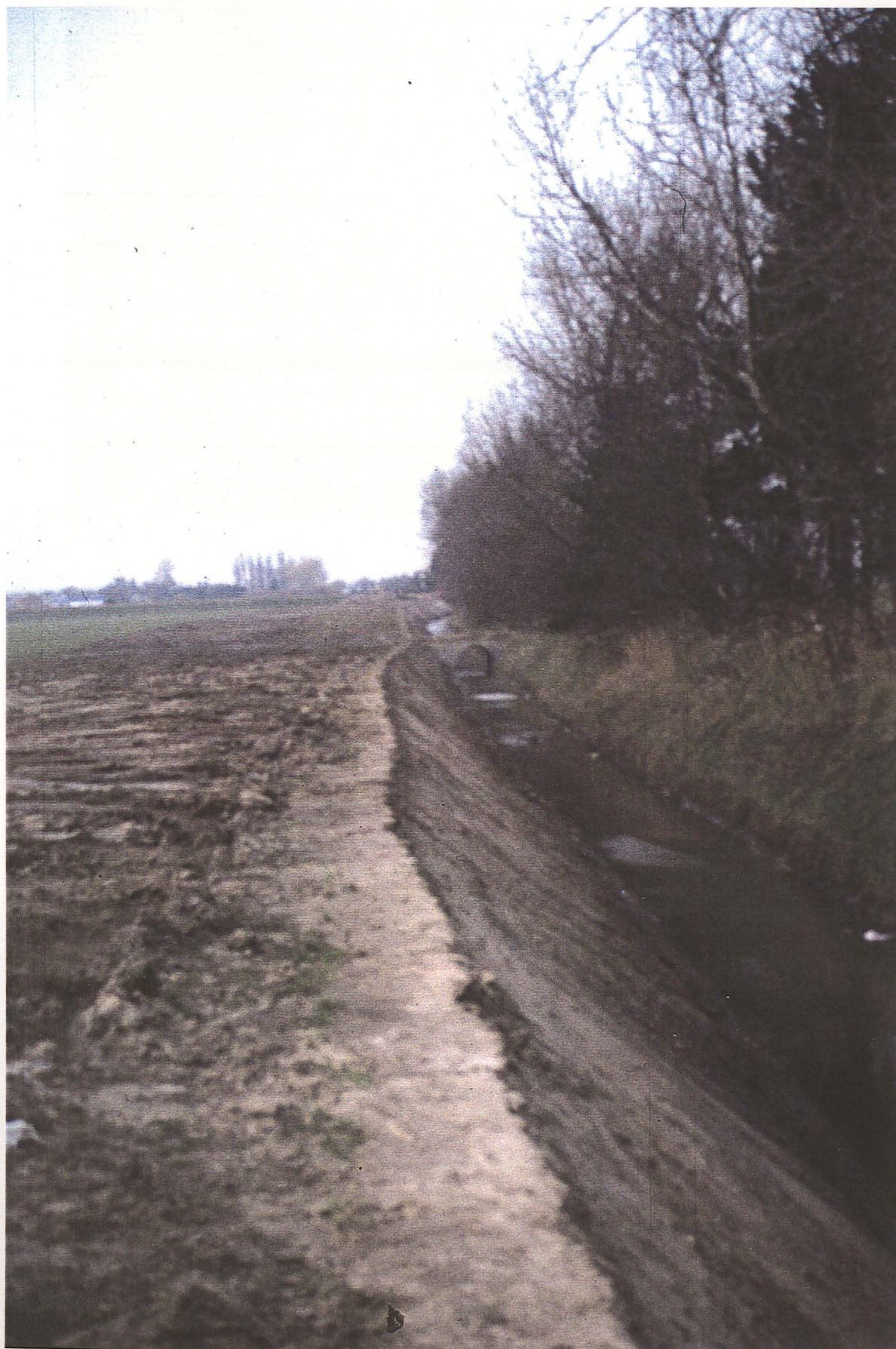
Plate 1 General View of Pennygate Drain
