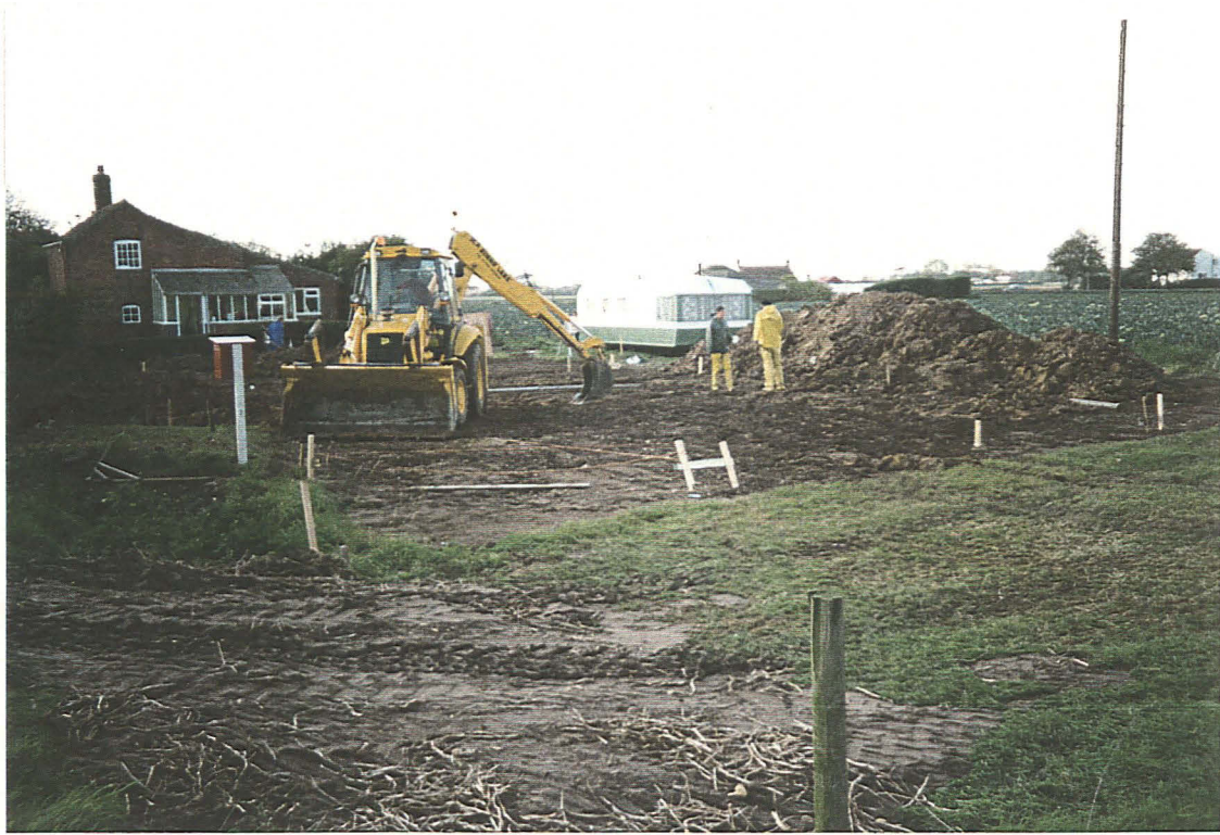
Plate 1: General Site View
