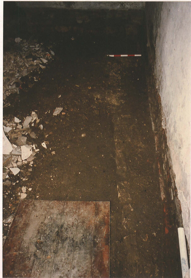
Pl. 13 Stone slab, 10, foundation beneath partition wall.
