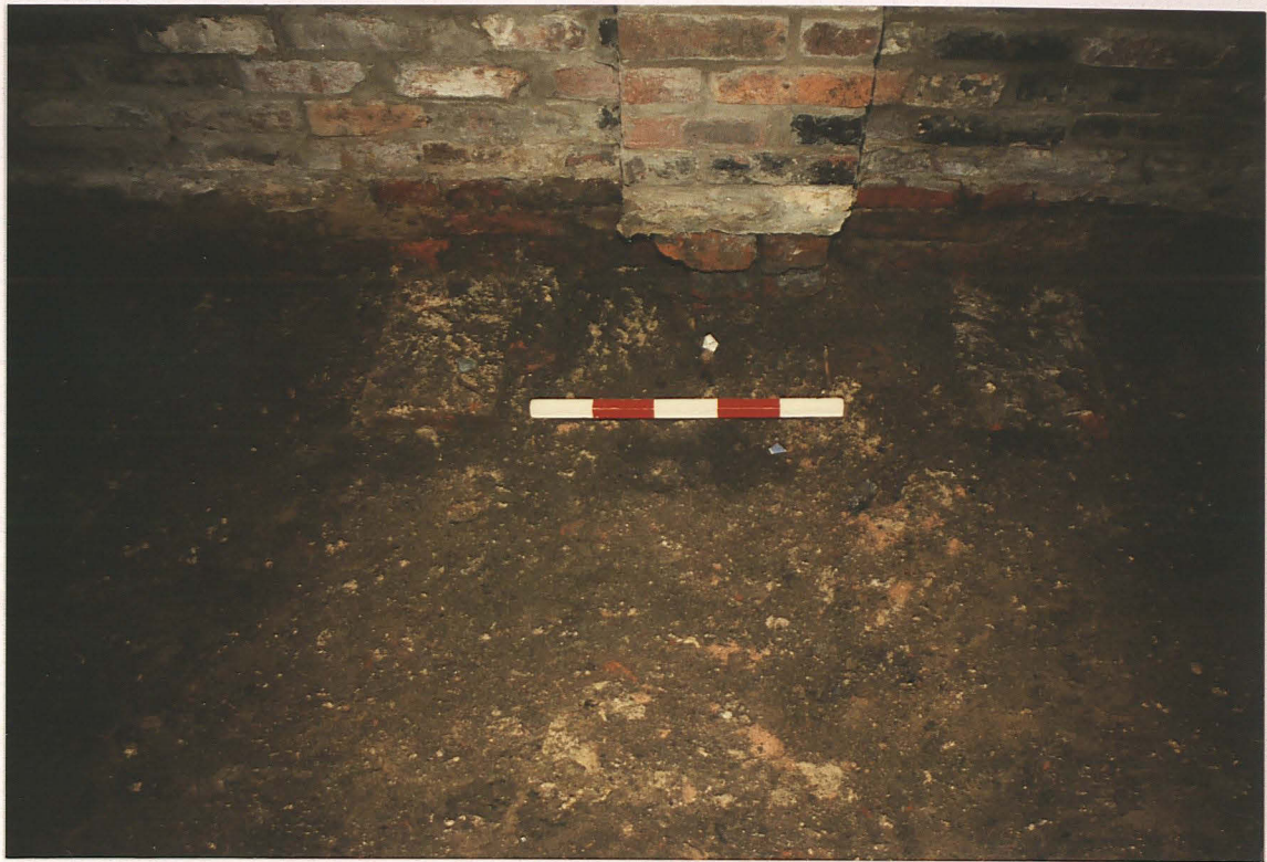
Pl. 9 Close-up view of brick supports, 22, for fireplace or copper boiler.
