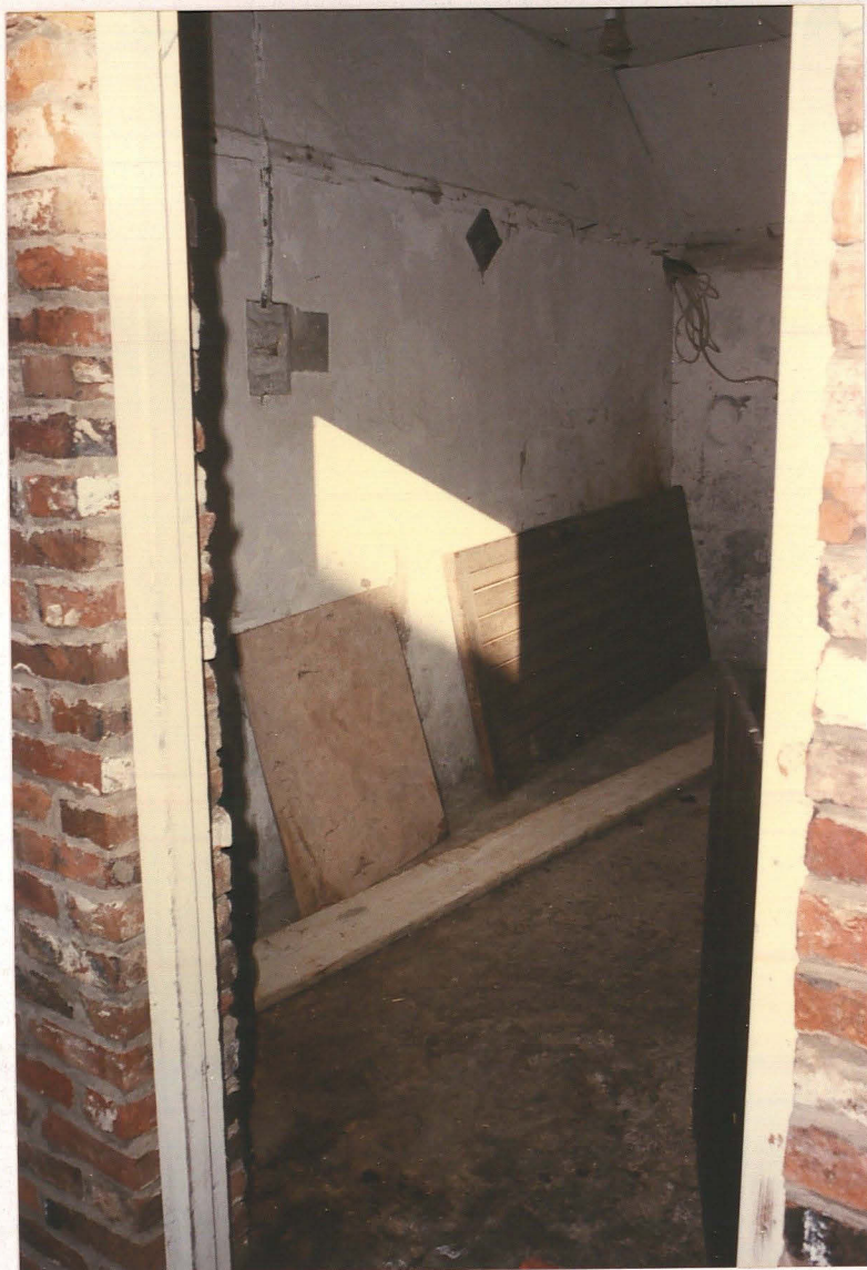
Pl. 11 General view of east bay and partition wall.
