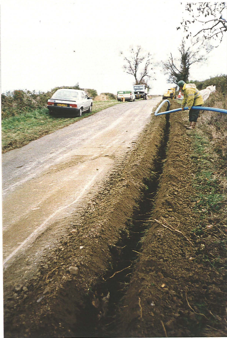
Plate 1: General Site View
