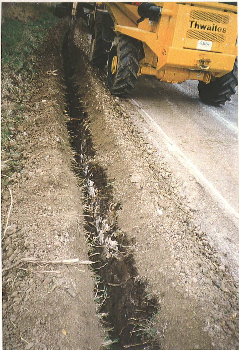
Plate 3: Stone Layer/Foundation (005), section 3
