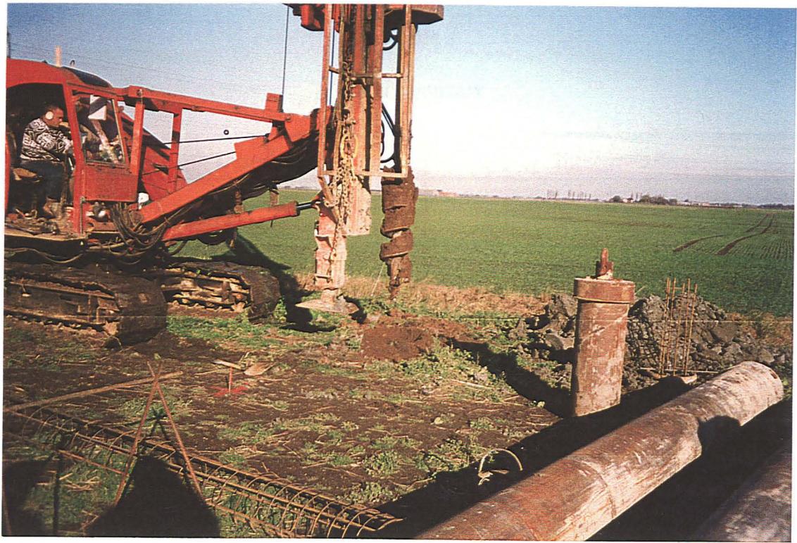
Plate 1: General Site View
