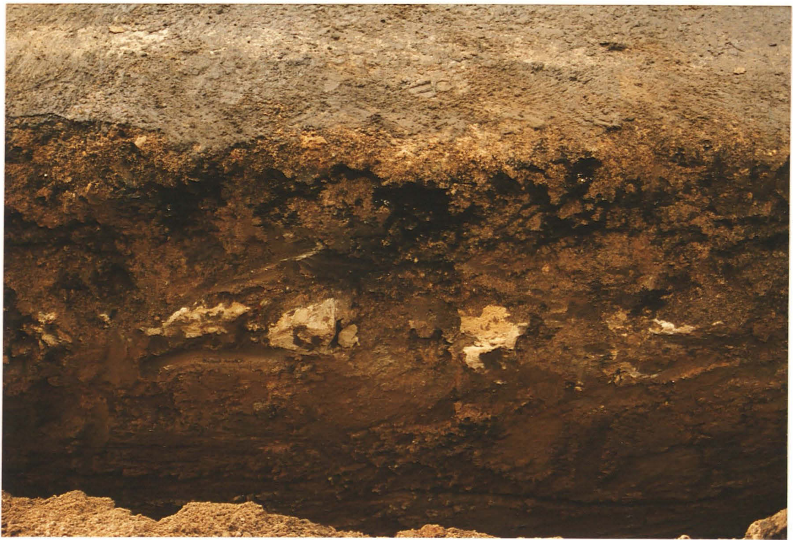
Pl. 3 Chalk rubble blocks 3 of the post-medieval Caistor to Market Rasen road, visible beneath the modern A46.
