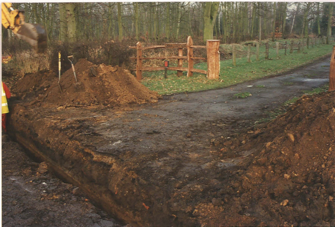
Pl. 5 The pipe trench across the Wood Cottage track, showing the thin upper lenses above a cambered rubble road 3 (looking NE).
