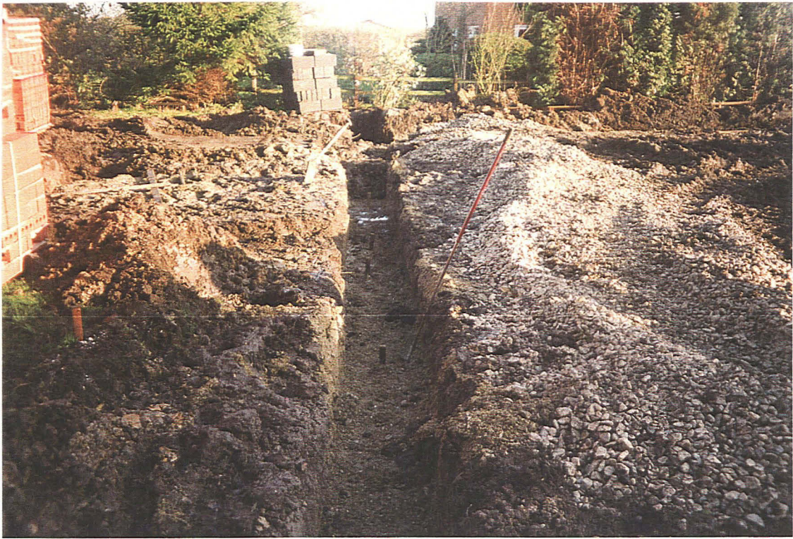
Plate 1: General Site View
