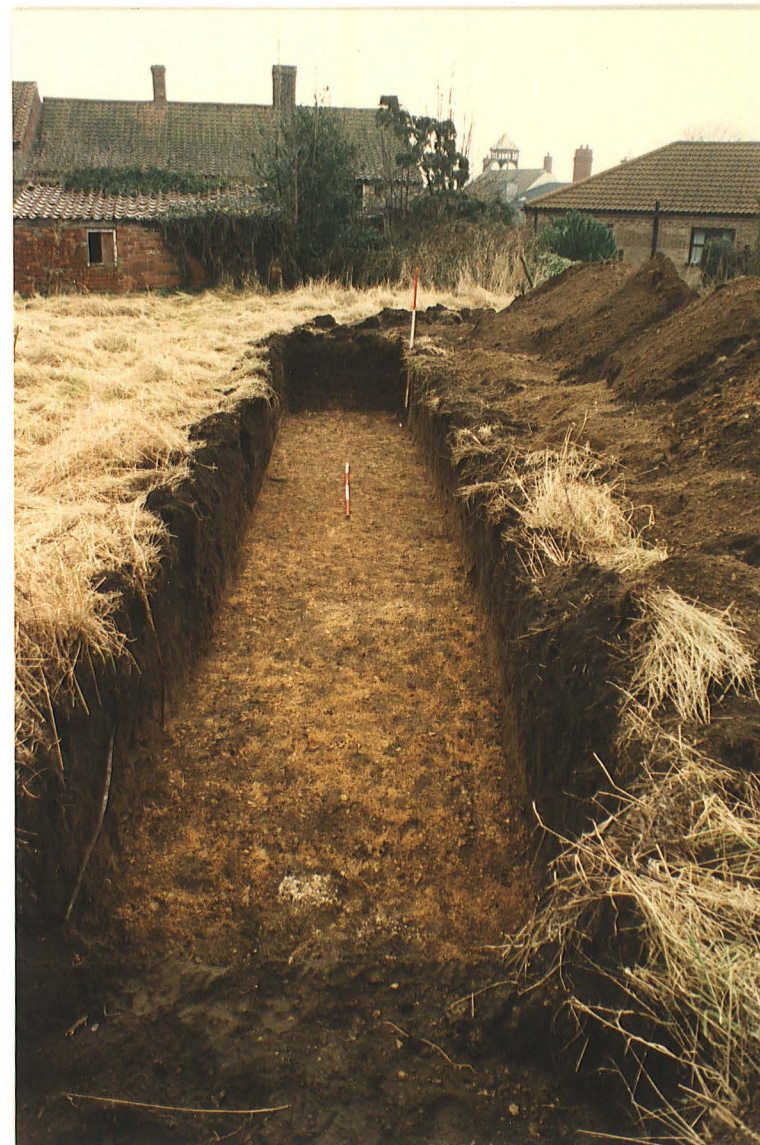
TRENCH 1 Looking South
