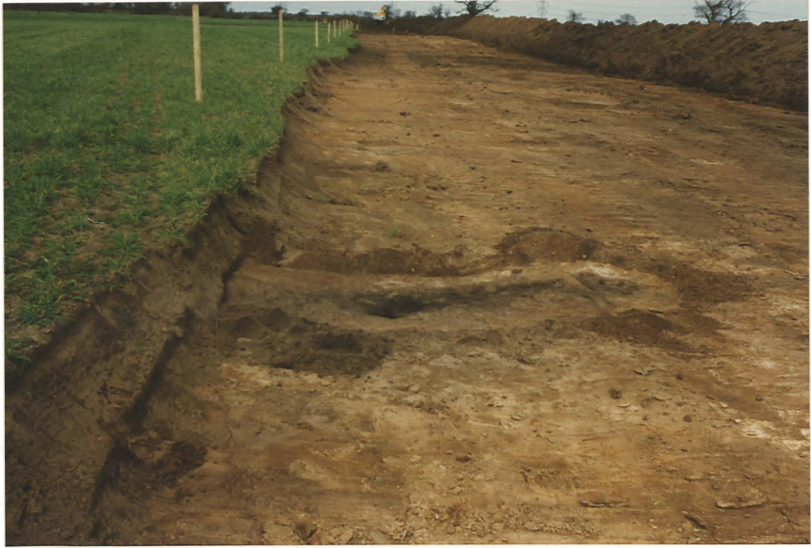
PI. 39 The pipeline easement, Field 12, after topsoil stripping. The darker soil (middle distance) was interpreted as a post-medieval ditch but may have been the return of the Iron Age enclosure ditch. (Looking north from gully 101).
