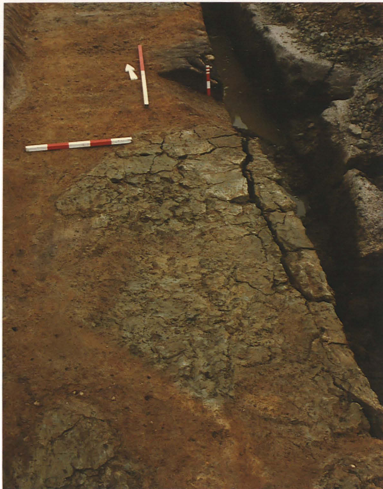
Pl. 25 Large sections of the new trench sides cracked and slumped within days; this process replicated events when the Iron Age ditch was dug. (Looking north past ditch terminal 307).
