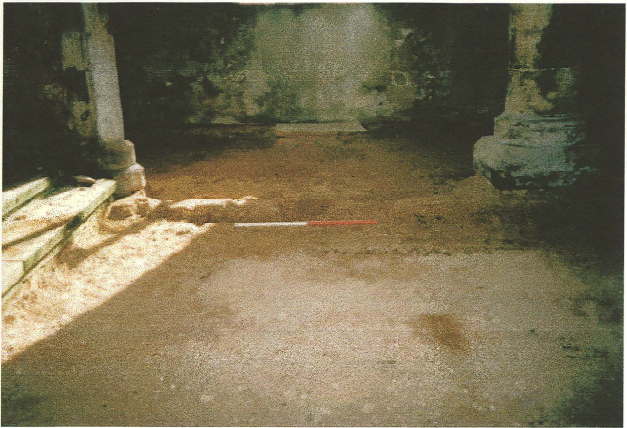
Plate 3 : Early wall, underlying columns of the south arcade. Note possible floor surface (foreground).
