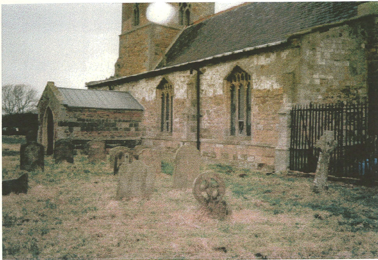
Plate 1 : General view, showing south porch.
