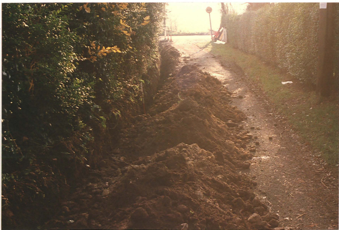
Pl. 6 In Orchard Road, large rounded pebbles forming a metalled surface were seen in the trench face 8 (looking south).
