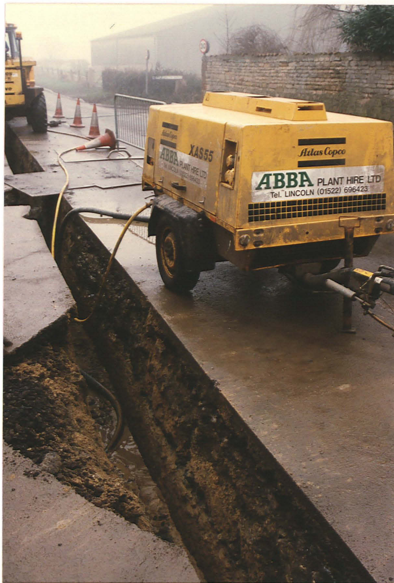
Pl. 1 Trenching along Reepham Road close to Blacksmith Road (looking east).
