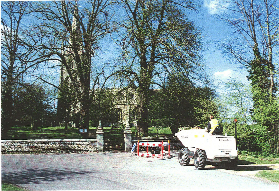
P1. General view showing location of Pit 1, looking north
