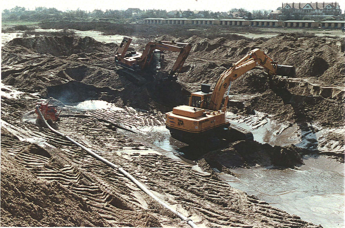
P1. General view of excavation work in progress (note flooding)
