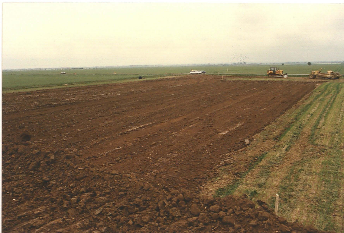
Plate 4: Site after being topsoil stripped, looking south-west
