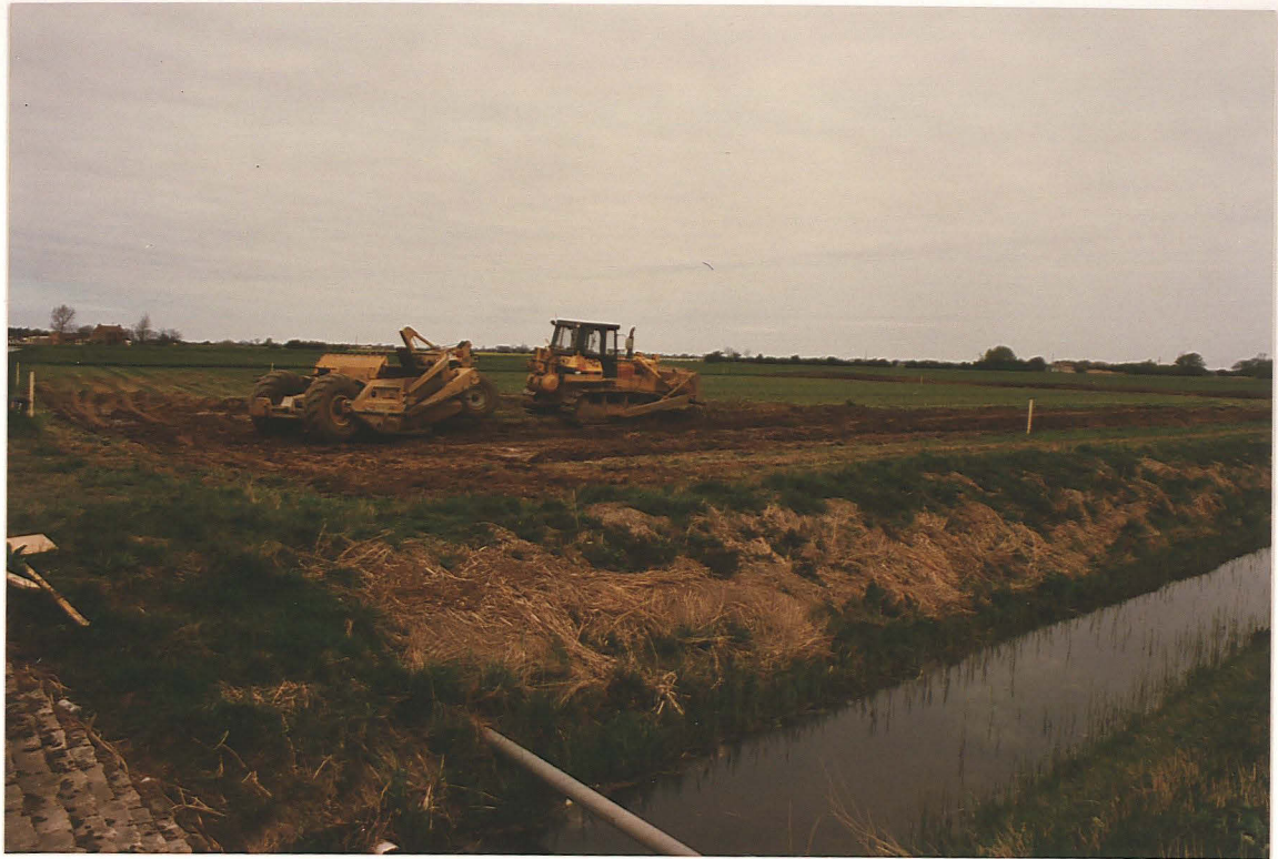
Plate 1: Topsoil stripping in progress, looking north
