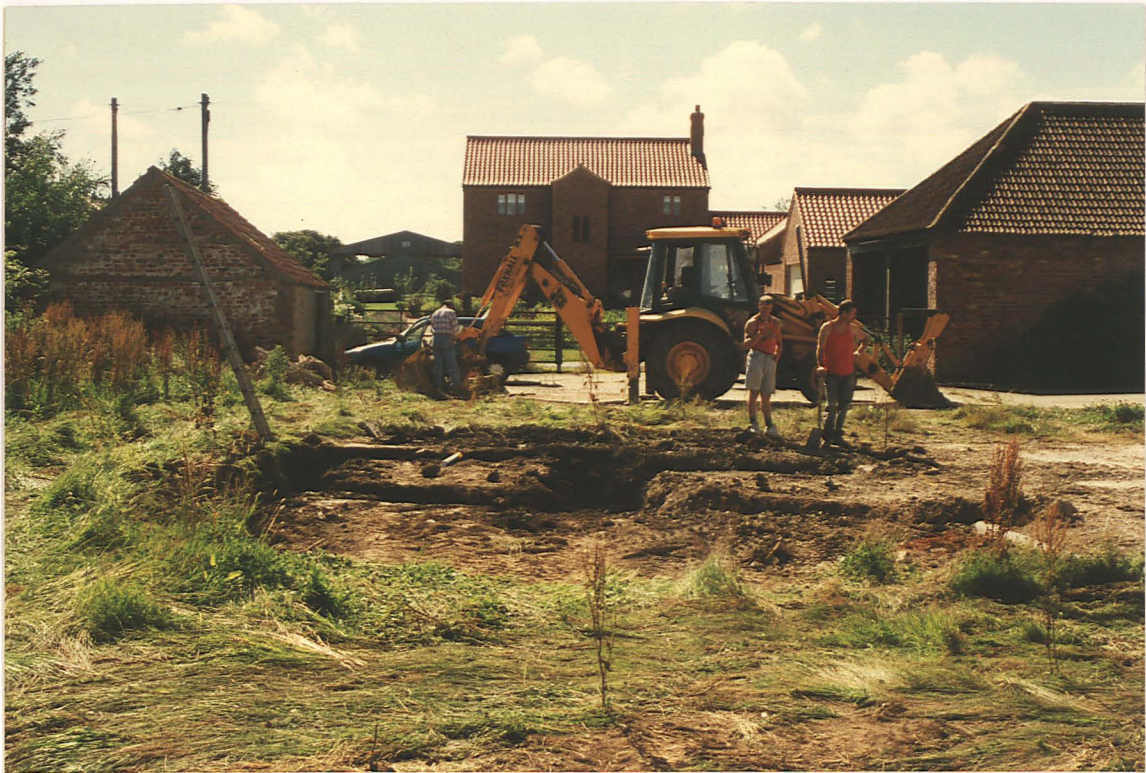
Plate 1: General Shot of site looking south
