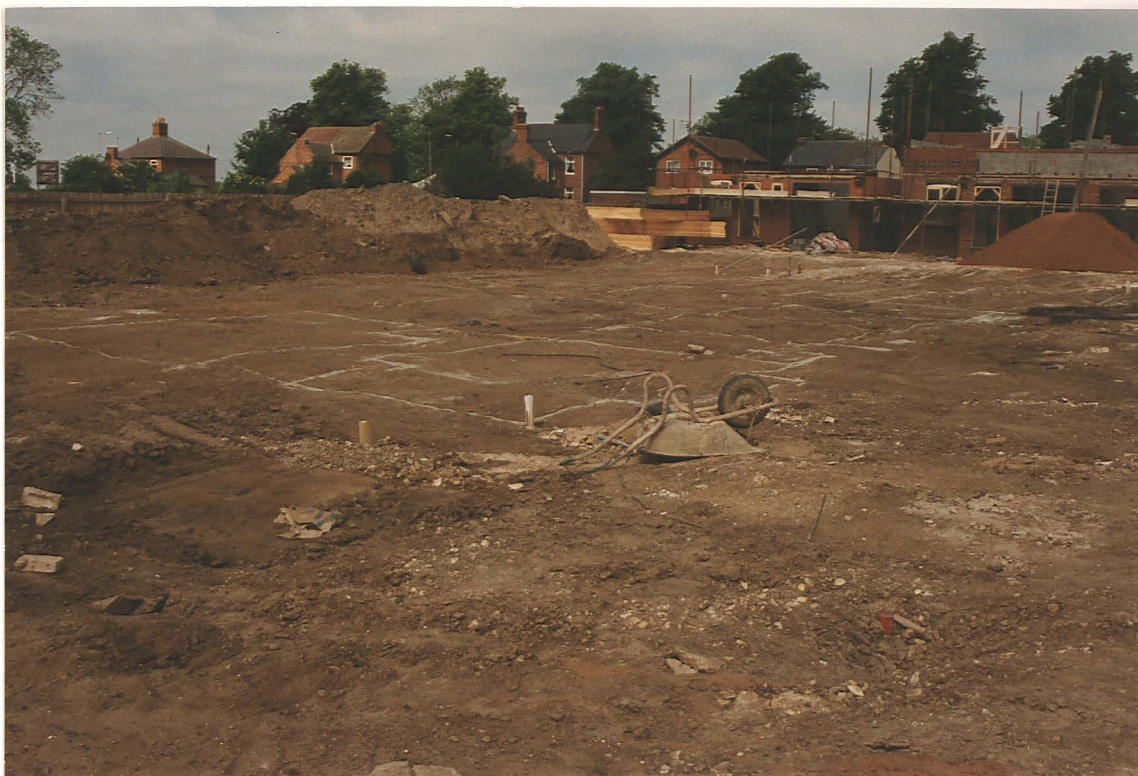
Pl. 1 Site of the monitored house foundations (looking NW).
