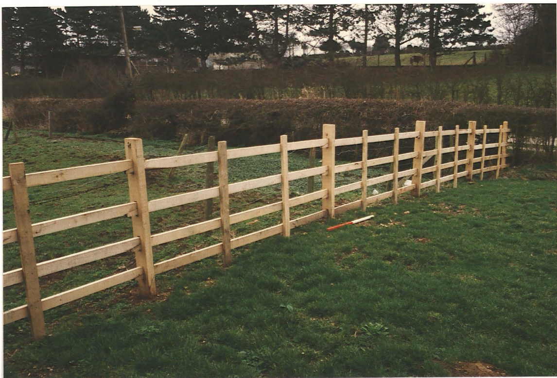
Plate 4: Eastern boundary fence completed, looking south-east.
