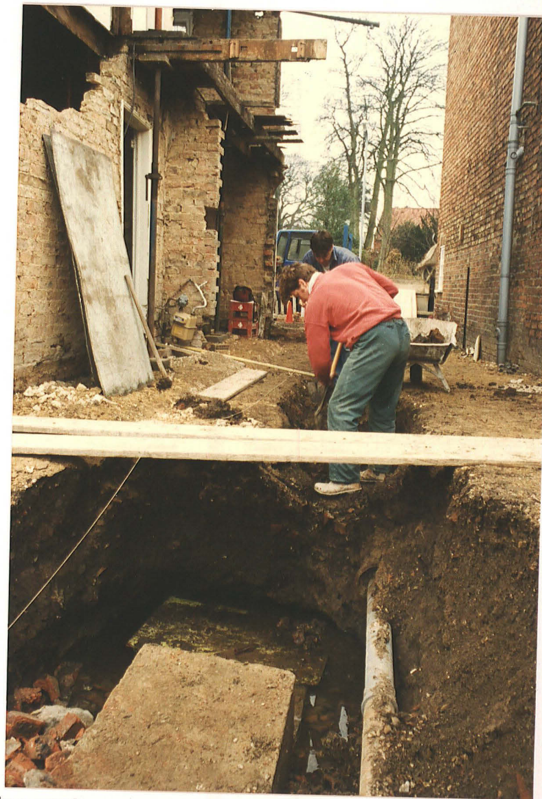
Plate 2: General shot of the excavation looking west
