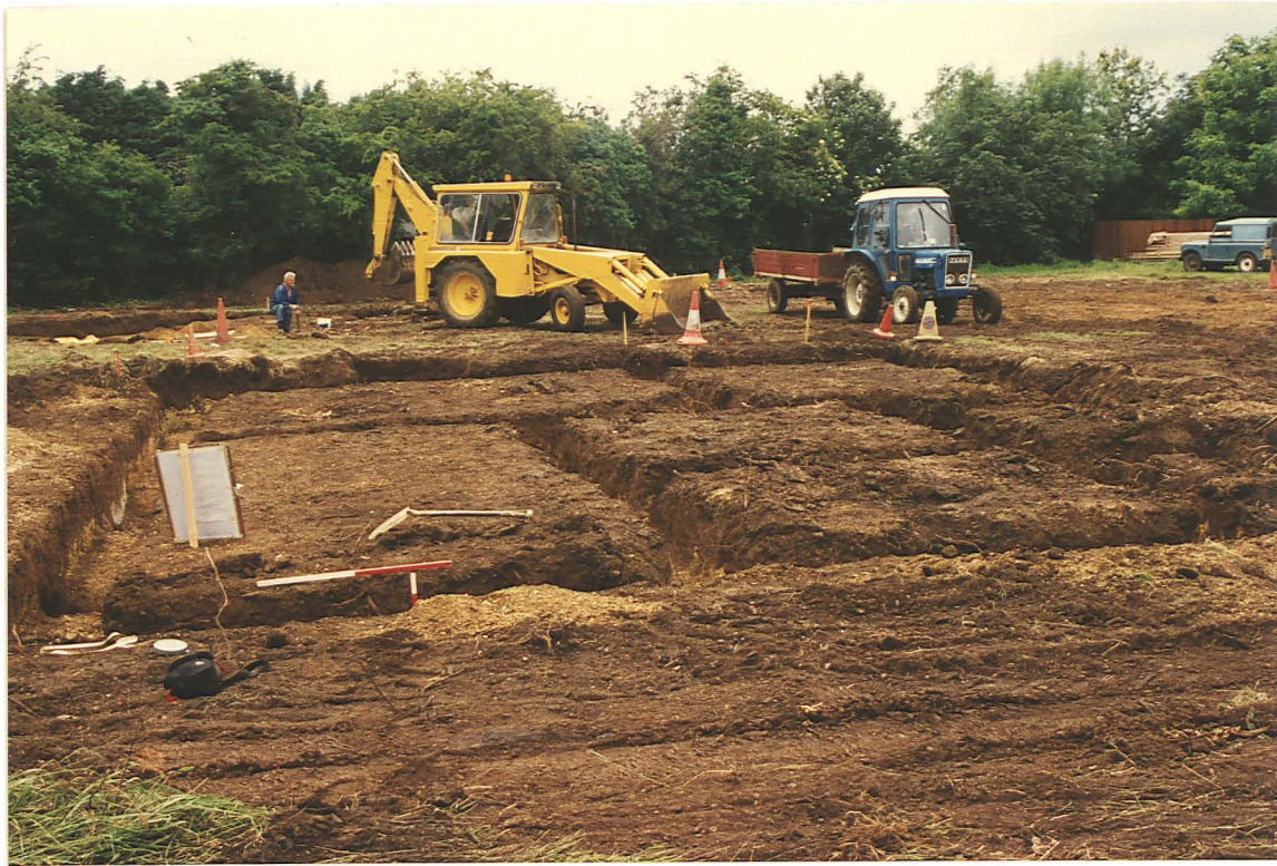
PI 1 General view of the foundation trenches in house plot 1.
