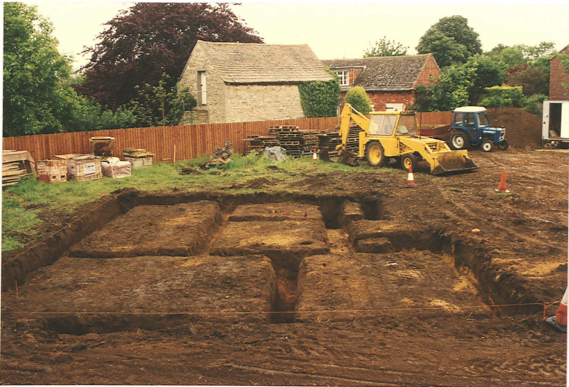
PI 14 General view of the foundation trenches in house plot 3.
