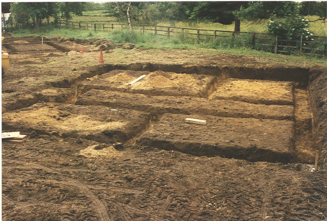
PI 8 General view of the foundation trenches in house plot 2.
