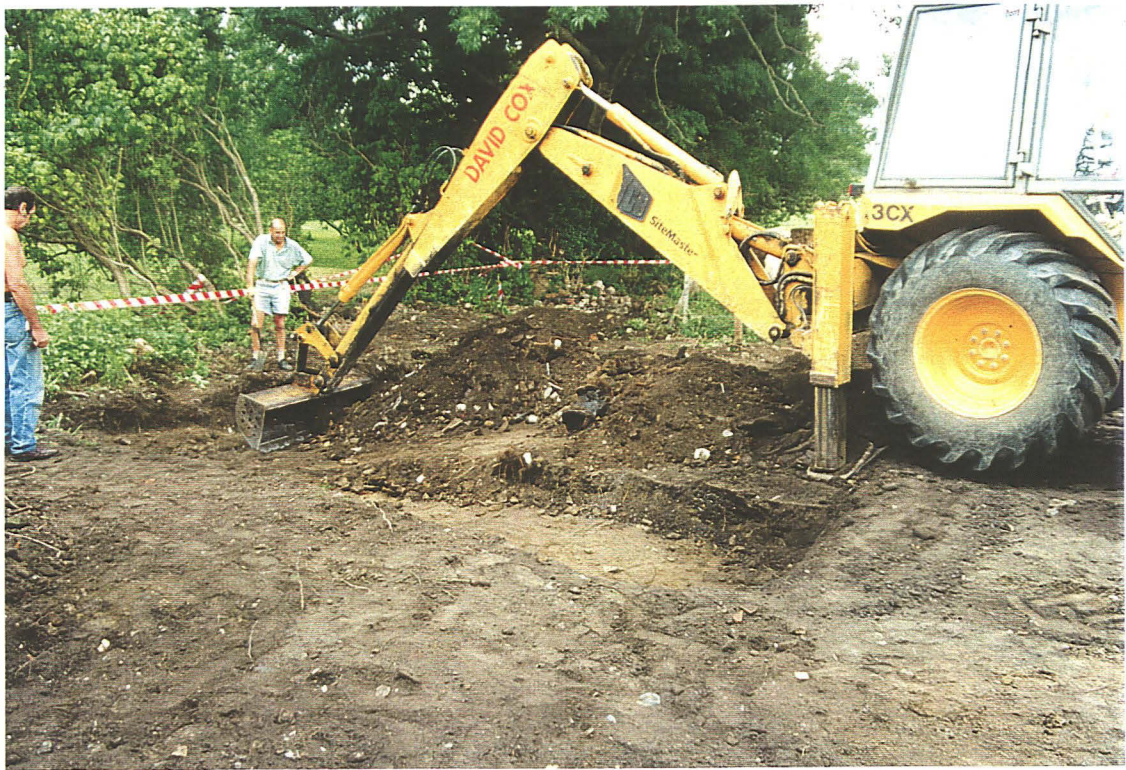
Plate 1: General shot during excavation of garage raft foundation looking north-west
