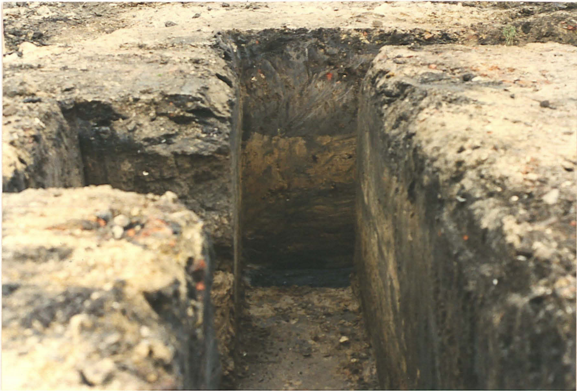
PI 5: East facing section of the south western corner of the foundation trenches, showing the sandier layers on the western side of the site.
