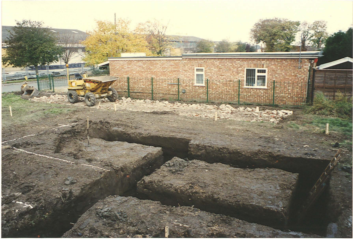
PI 1: View of the site, looking north.
