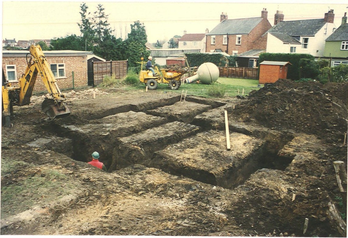
PI 3: Excavated trenches, looking north east.
