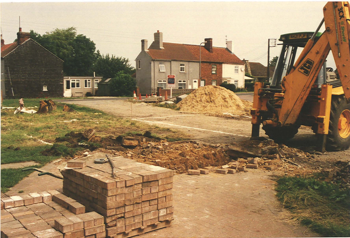
Pl. 6 Excavation of footings for house plots 3 and 4 (looking north).
