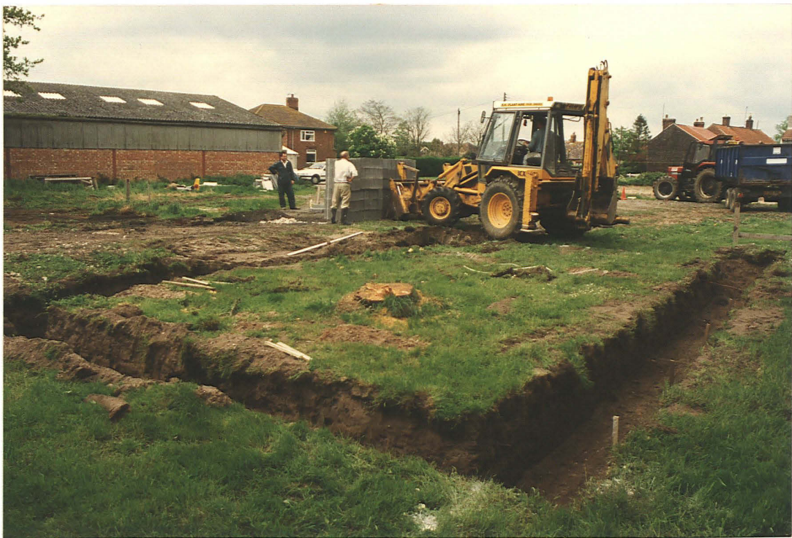
PI. 2 Excavation of footings, plots 9 and 10, looking NW.
