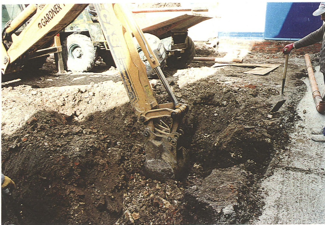
P1. Excavation of an internal wall trench through [104] showing the loose nature of the deposit. Looking north-west.
