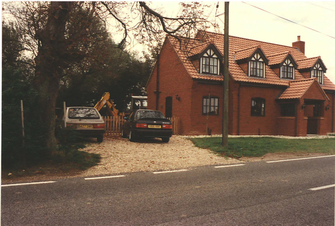
Pl. 2 Temporary fence to garage site. Moat inner bank approximately level with ground floor window glazing bar. From north.
