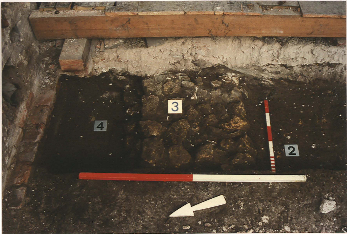
Pl. 5 Wall 3 and deposits 2 and 4. Note foundation off set. View ESE. Scales 0.50m and 1m.
