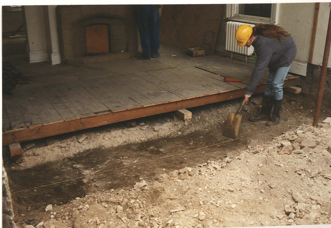
Pl. 2 Initial cleaning of the foundation trench. Looking SE.
