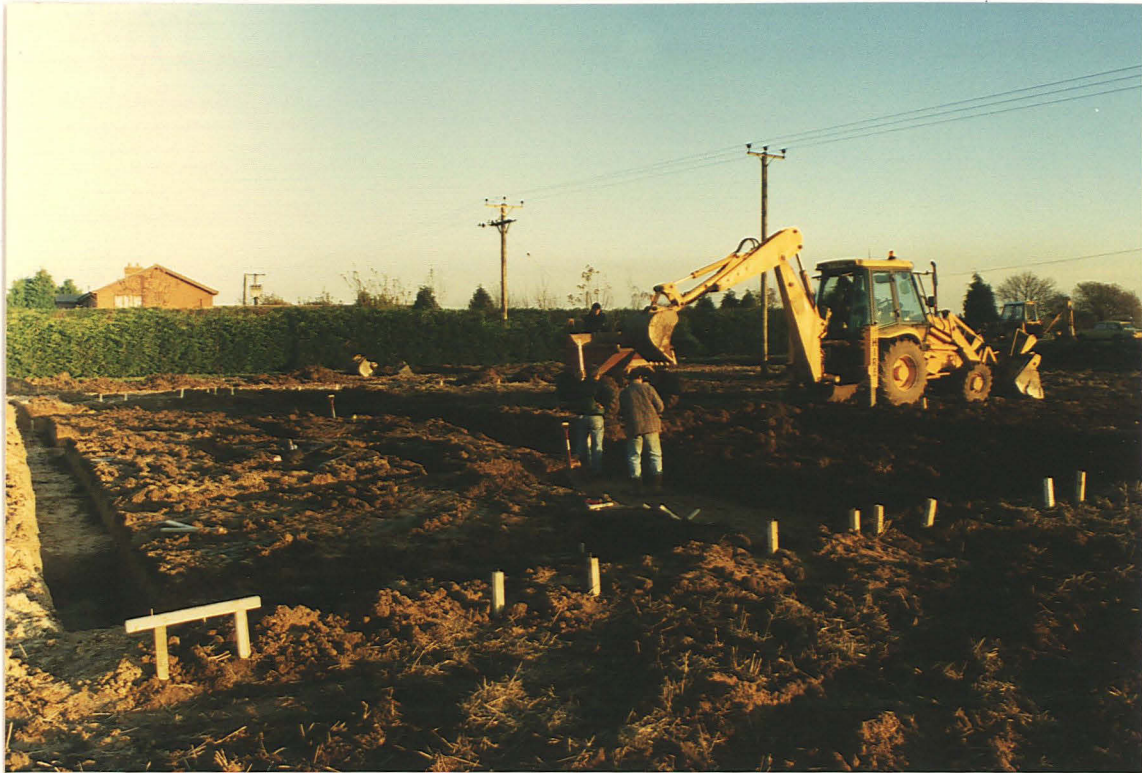
Pl. 1: View of excavated foundation trenches, from north-west corner, looking south-east.
