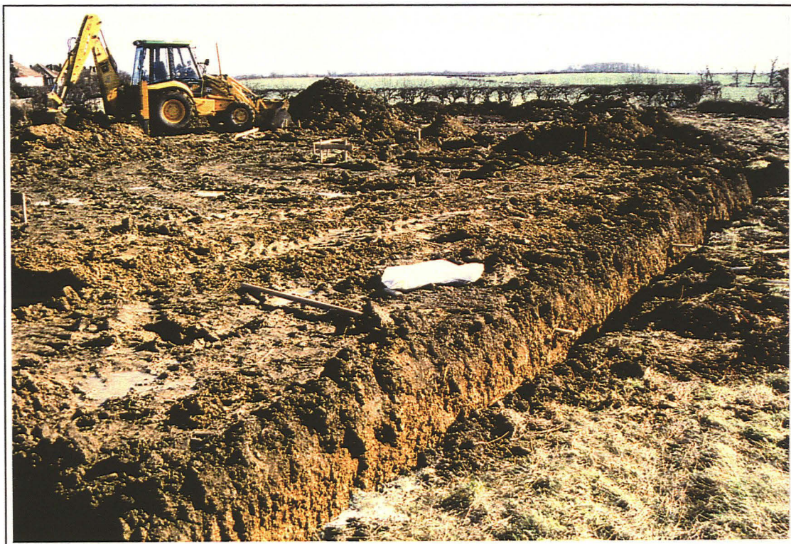
Plate 1: General view of Plot 1 looking east, showing mechanical excavation of foundation trenches.
