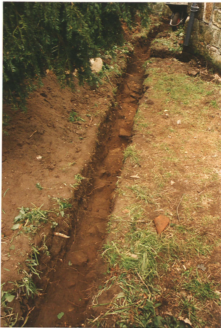
Pl. 9 Trench 3 west of Trench 4 showing sandstone foundations
