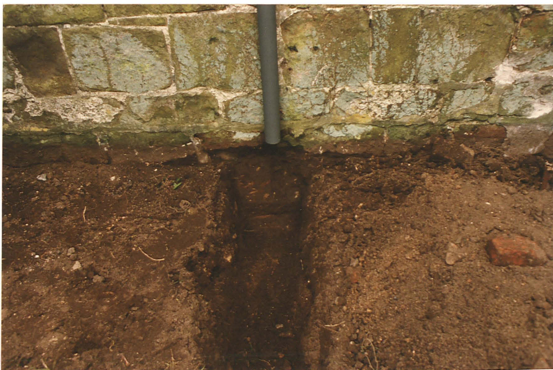
Pl. 2 Trench 6 at junction with tower north wall showing chamfered plinth
