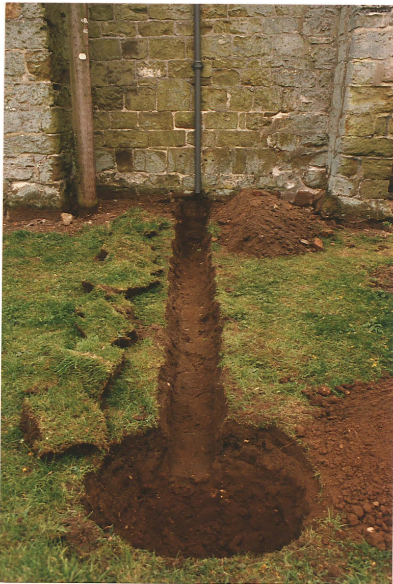
Pl. 1 Trench 6 and soakaway running north from tower
