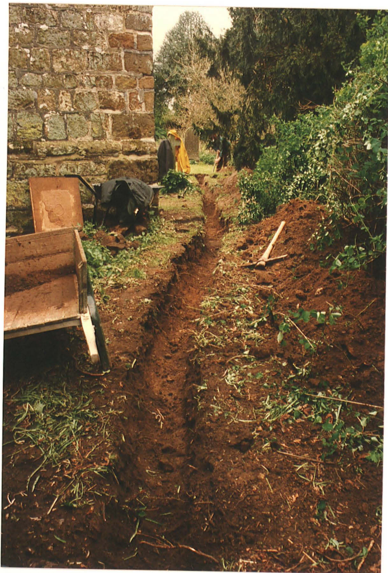
Pl. 7 Trench 3 to north of chancel looking north-west
