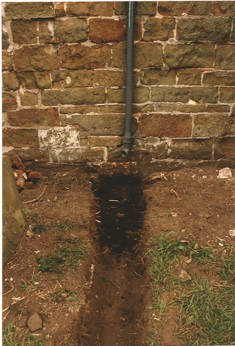
Pl. 4 Trench 1 at junction with tower south wall showing chamfered plinth
