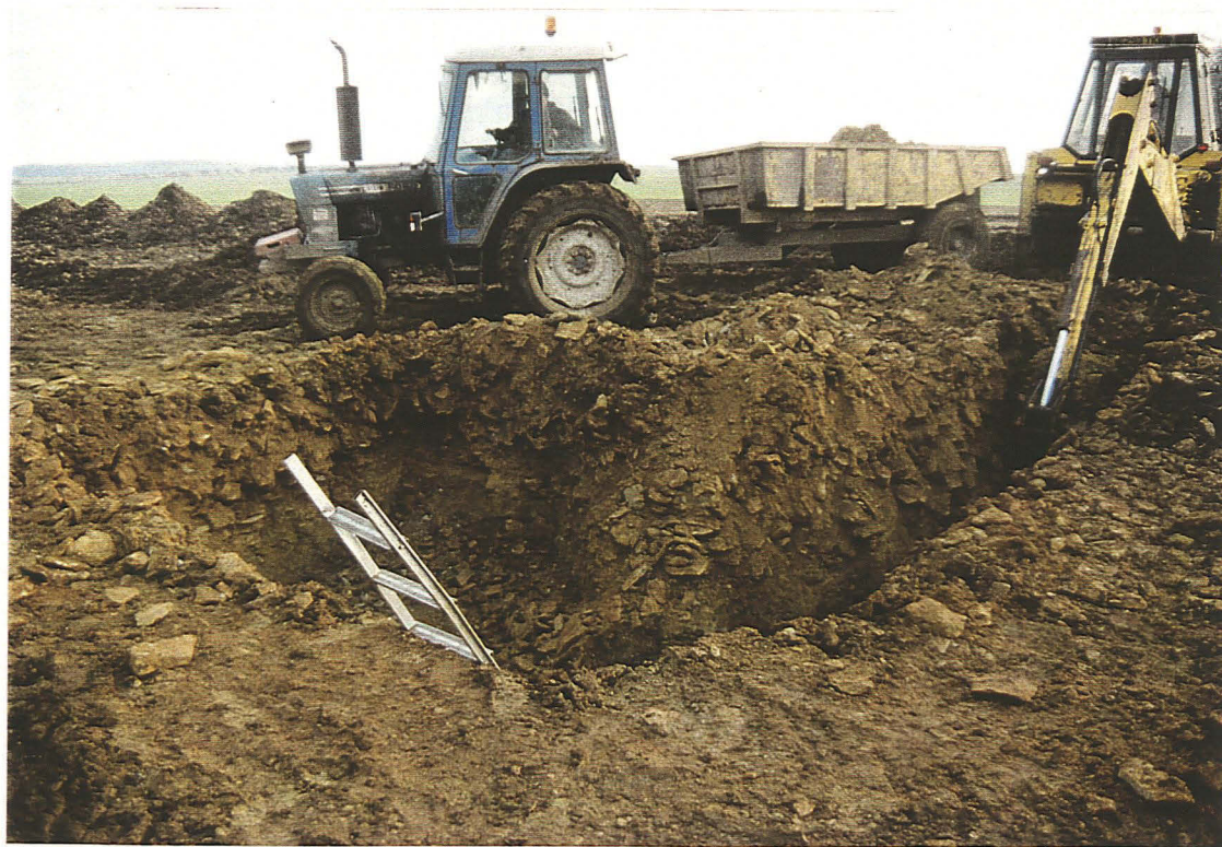
P2 Excavations of waste tank in progress, looking south-east
