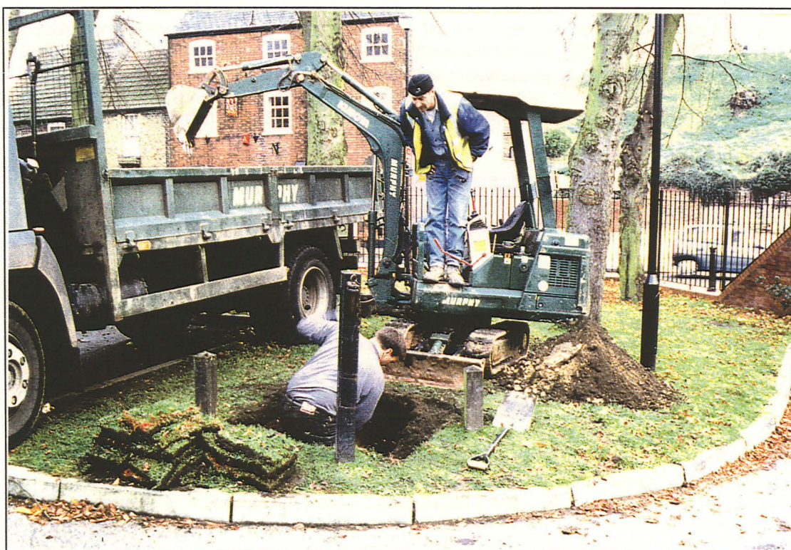
Plate 1: General view showing contractor's excavation of Trench 1 looking east.
