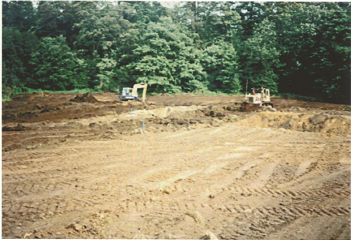
Plate 1 : General view of site, looking north east
