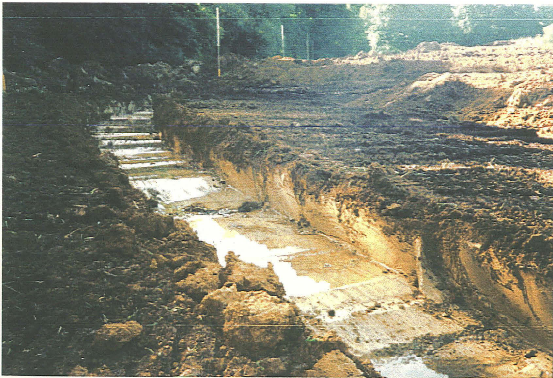
Plate 2 : Machine dug drainage trench around perimeter of lagoon
