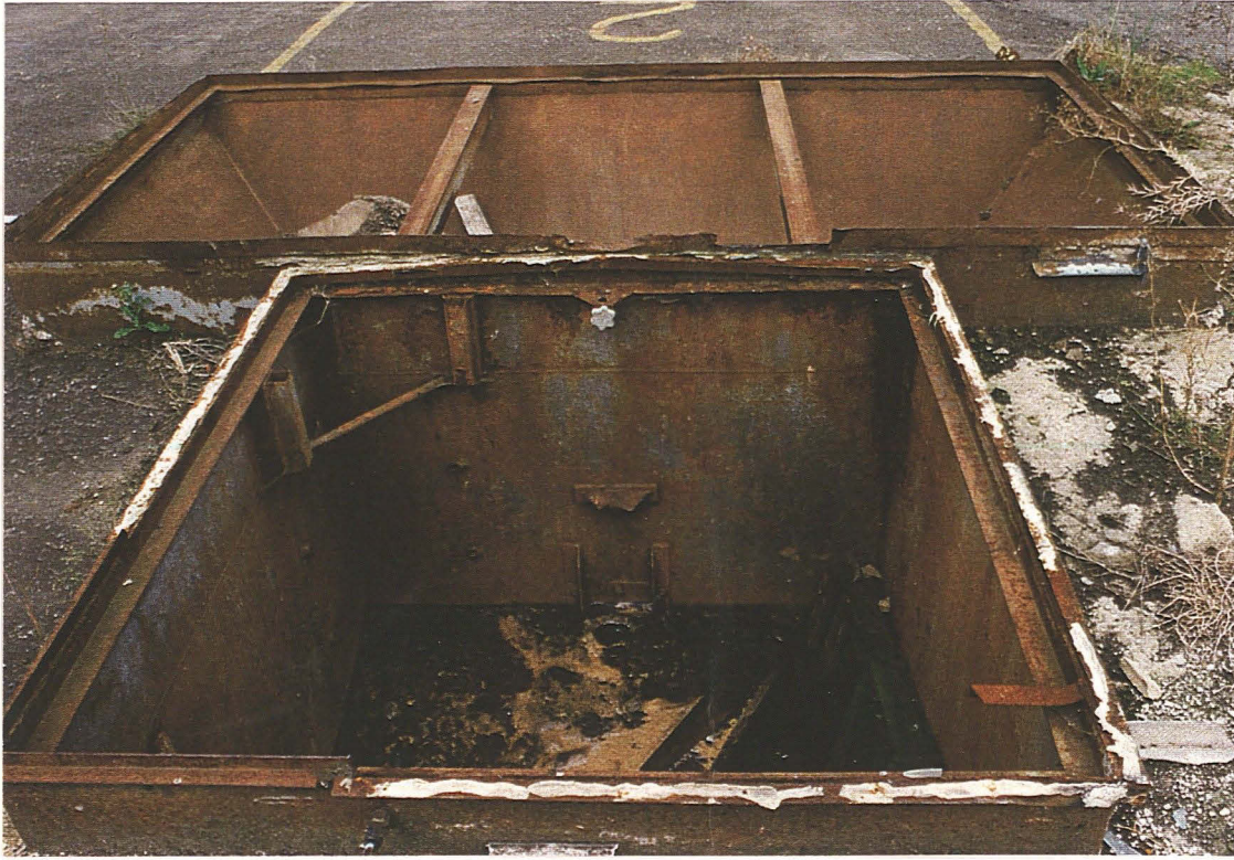
Pl. 3 Underground storage tanks.
