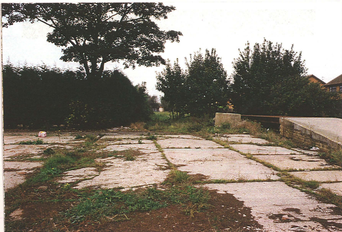
Pl. 2 Concreted area at western part of the site.
