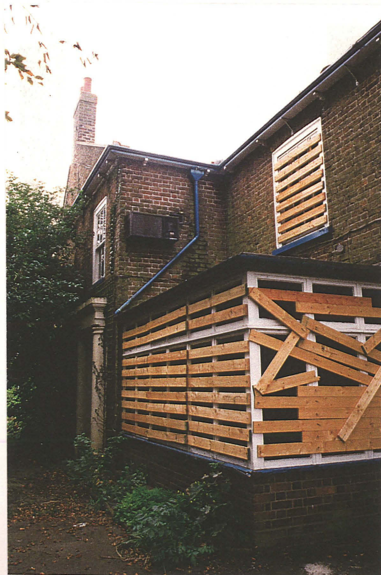
Pl. 6 North-east corner of Phoenix House showing 20th century extension.
