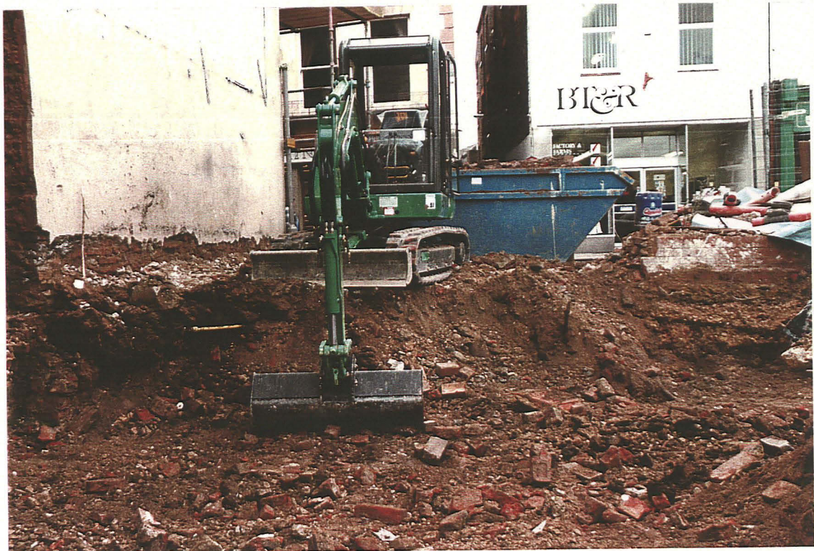
P1. General view of foundation footprint during machining, looking west
