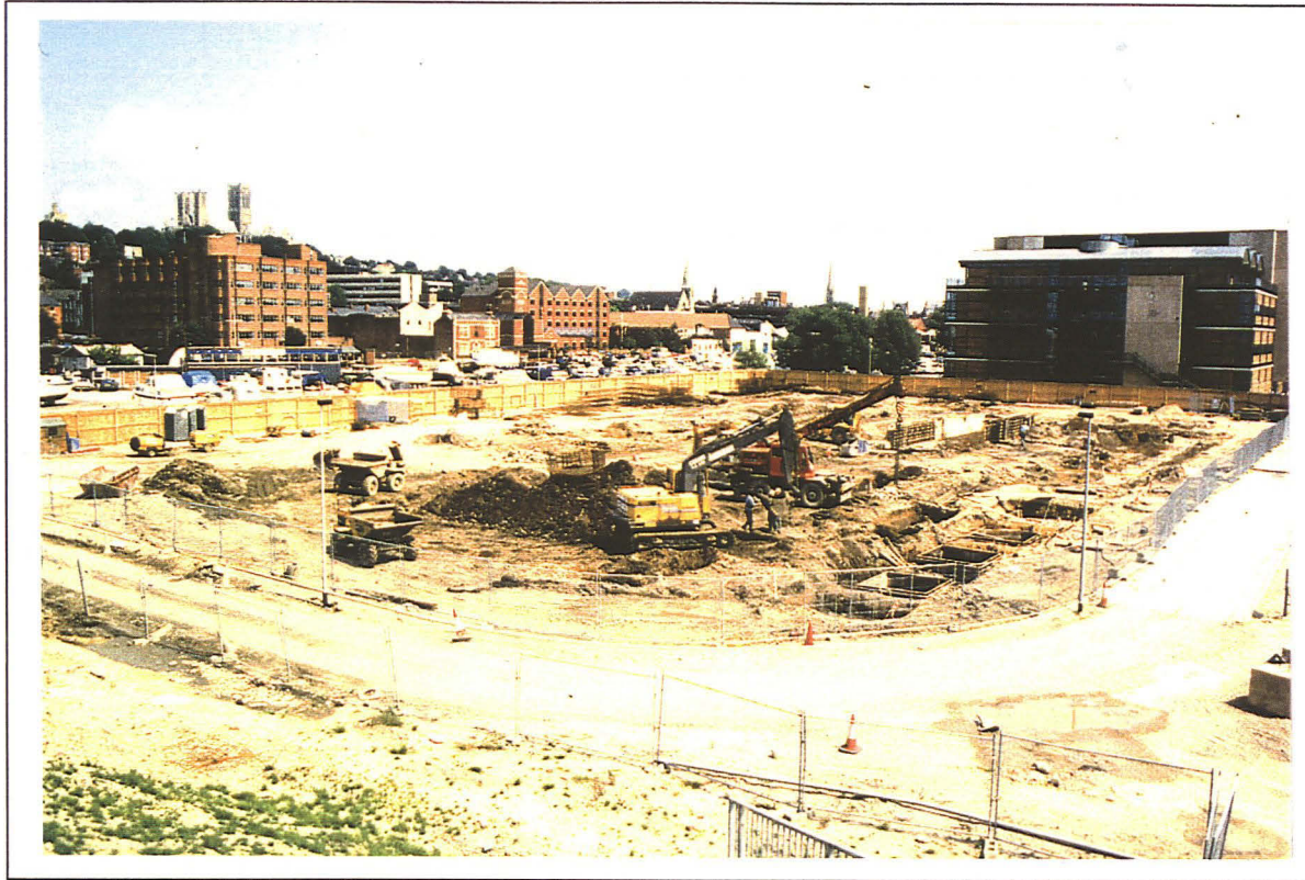
Plate 1: General shot of site during construction
