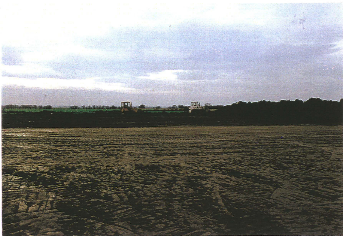
Pl. 2 Topsoil stripping in progress.
